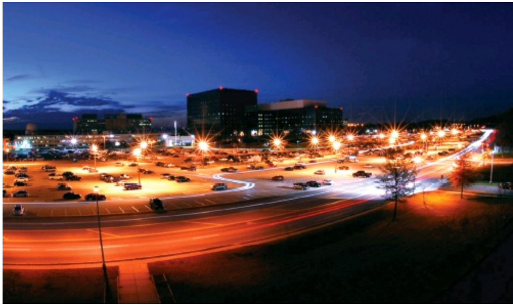
The National Security Agency, the nation's eavesdropper, never sleeps. NSA buildings in Maryland total 18.6 million square feet of space, 1.3 times the size of the Pentagon. (Sandra McConnell, NSA)
