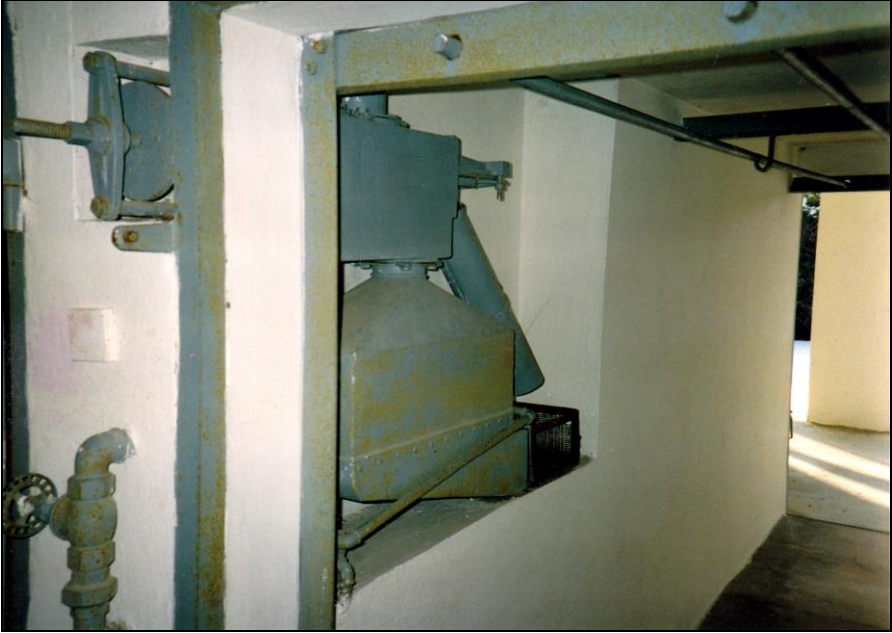
Document 46: Degesch circulation device in one of four Zyklon-B disinfection chambers at the Dachau Crematorium in 1990. © Carlo Mattogno.
