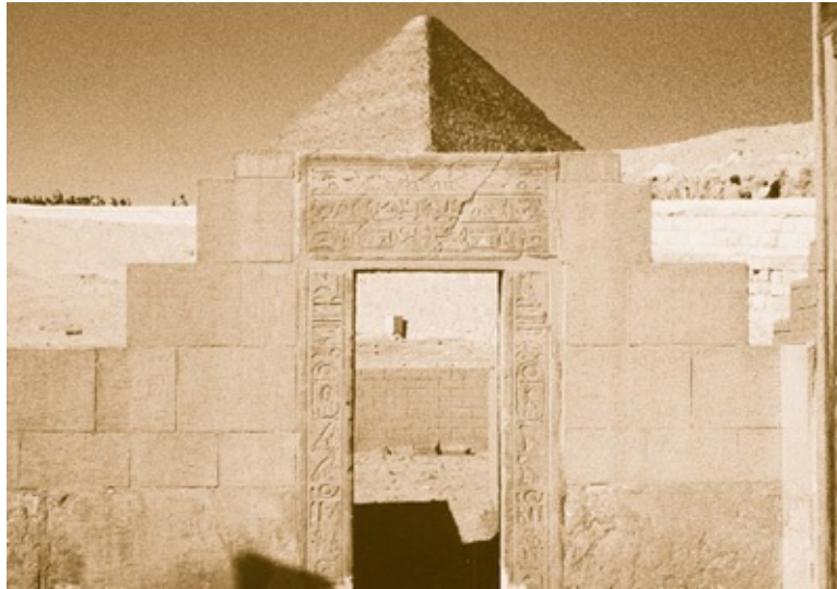
Figure 7.3. This interior doorway of the small New Kingdom Temple of Amenhotep II at the northeastern corner of the Sphinx Pit has been constructed in such a way that it is in perfect alignment with the Great Pyramid, whose apex is aligned with the center of the doorway and lintel. The view is toward the northwest. The wall beyond the temple, where some people are, is the foundation and border wall of the modern access road from Nazlet el-Samman to the pyramids. It was constructed some time after the Second World War. The siting of this temple in such an obvious way to align with the apex of the Great Pyramid reminds us of the relationship of the apex of the Pyramid of Chephren with the floor of the Sphinx Temple (that sight line is at the golden angle, as measured with an inclinometer), and also the general Giza Plan, as it specifies the precise size and location of the Sphinx with relation to the two main pyramids, as described in the text. (Photo by Robert Temple)
