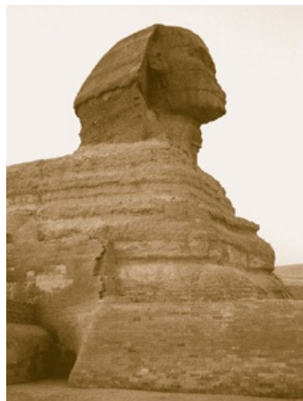
Figure 2.30. At dusk, when the glare of the sun has subsided, a clearer view is possible of the contrasting materials that now make up the outer surface of the "restored" Sphinx. Here we see that the elbow of the Sphinx is entirely covered in small modern
