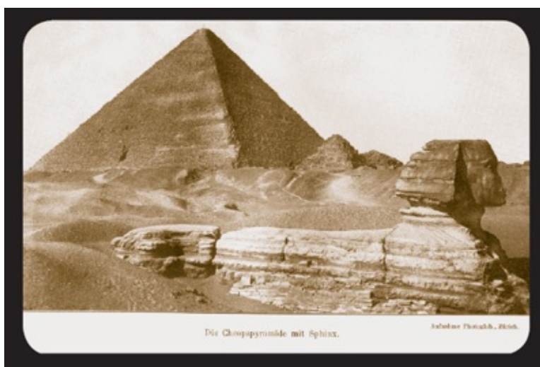
Figure 1.31. This photo, published in 1921, just a few years before Baraize filled it full of cement, shows clearly the cleft separating the main portion of the Sphinx from its rump. The rump had by this time split away due to the structural weakness in the stone caused by the hollow shaft that led down through the entire body of the Sphinx to the burial chamber beneath it at that point. The shaft was not original, but a later intrusion to enable a pharaoh to be buried in a chamber beneath the Sphinx, possibly a Saite pharaoh of the Twenty-sixth Dynasty, the last native Egyptian dynasty (664–525 BC). The Saites were obsessed by the Giza Plateau, and as part of their restoration efforts they may have partially or wholly cleared the Sphinx of sand, or at least cleared enough to give them ready access to the back so that they could make the shaft. By 1926, Baraize had entirely obliterated this evidence and permanently filled in the shaft with cement, thus making access to the subterranean chamber impossible. The rump tunnel inside the Sphinx also now terminates at this point, where Baraize's cement oozed into the tunnel and blocked it too. How far the lateral tunnel may have extended forward into the Sphinx's body, past the cleft and toward the chest, cannot now be determined. This photo appeared as a frontispiece in a rare volume that is not to be found in either the British Library or the Library of Congress, Die Cheopspyramide: Ein Denkmal mathematischer Erkenntnis (The Cheops Pyramid: A Monument of Mathematical Knowledge) , by the brilliant Austrian engineer Klaus Kleppisch, who lived in Warsaw. (Verlag von R. Oldenbourg, Munich and Berlin, 1921; collection of Robert Temple)
