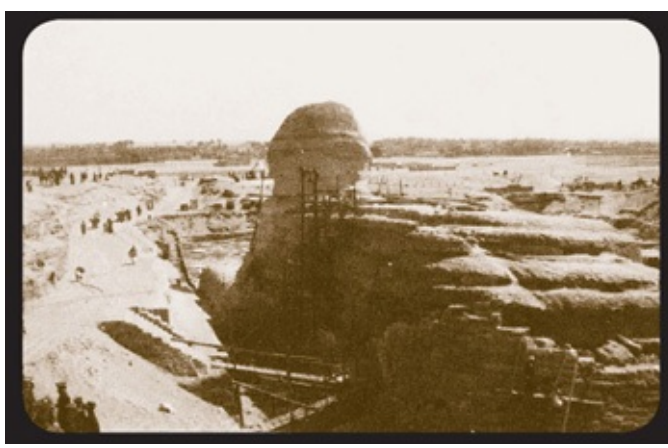
Figure 2.15. This snapshot was taken by a British tourist in 1936, during the excavation and restoration of the Sphinx by Selim Hassan. This is the only known photo showing the rear of the Sphinx during this period. It shows the fantastic extent of the erosion of the natural stone of the Sphinx's rump, and reveals that Hassan was collecting fallen blocks of stone and "reconstructing" the rump with them to such a depth that the rump as we see it today protrudes by perhaps as much as 10 feet from the actual underlying stone itself. At the top of the ladder at the rear in this photo is a platform made of replaced stones big enough for at least a dozen people to stand on! Nowhere in his excavation report does Hassan mention that he did anything like this. To the left in the photo are the modern walls constructed by Baraize in 1926 to hold back the sand on the north side. Although he later demolished these, at this stage in his work Hassan was using them to anchor his planking gangways for his workmen to get across to the body of the Sphinx. It is believed that no other photographic evidence of any of this work exists, and this has never been published before. In the distance, it can be seen that the Sphinx Temple has not yet been excavated. ( Collection of Robert Temple )
