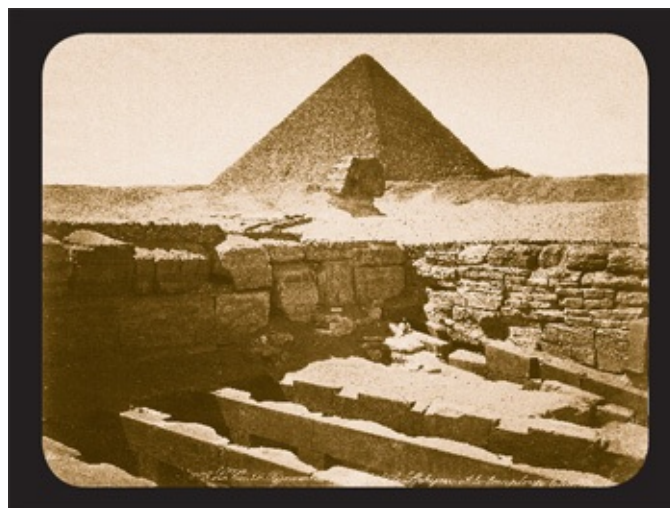
Figure 6.67. This old photo by Bonfils, probably dating from the 1890s, shows the Valley Temple sanding over subsequent to 1870, when its interior had been excavated by Mariette. Walls made of small stones closely hug the west wall (at rear in photo) and the north wall (right in photo). The Valley Temple during the period from the New Kingdom onward acted as a kind of sand-filled megalithic foundation for inferior structures of small stones and mud brick, which even in this photo have not been fully cleared away. It was only when Uvo Hölscher finally excavated the Valley Temple in its entirety and cleared its outer walls that all
