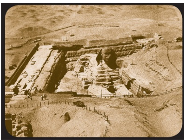
Figure 6.50. This is an aerial photo of the Sphinx taken by the British Royal Air Force on September 28, 1926 (as we know from the information on the back). This image has never been published, as far as I know. This is probably the best photographic evidence to survive of the gigantic barrage walls constructed by Baraize earlier in this same year to hold back the engulfing sand. As can be seen here, his major effort was to prevent the sand from pouring in from the north (on the right in this photo) and the east (the foreground in this photo), since the southern portion of the Sphinx Pit had been completely cleared by him and the portion of the Chephren Causeway beside it had also been cleared. It is remarkable that at this late date, the remainder of the Chephren Causeway was completely covered by sand and was invisible. This photo provides graphic evidence that the Sphinx Temple in front of the Sphinx was still completely unknown, covered in a vast hill of sand. Above and behind the Sphinx Pit, which has been cleared to the bedrock at the back, Baraize has erected strong walls to stop the sand pouring in from the west. All these overwhelming perils of sand were not eliminated until 1936, when Selim Hassan, with hundreds of laborers and railway tracks (see figures 3.11 and 3.12), finally carried it all away in one of the most Herculean clearance efforts in the history of world archaeology. At that time, in clearing the mountain of sand seen here in the foreground, he discovered and cleared the Sphinx Temple underneath, which had been lost beneath the sand and forgotten no later than 2000 BC (which was the end of the Old Kingdom period). This is one of the most historically important photos ever taken of the Sphinx, and I bought it from a dealer for only £2.99. Sometimes in life one gets a bargain. ( Collection of Robert Temple )
