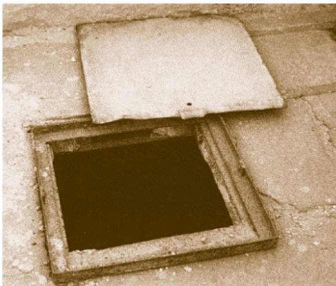
Figure 1.29. I lifted the lid and took this photo of the modern metal frame that has been inserted into the bedrock floor of the Sphinx Pit between the feet of the Sphinx. This is the entrance to the underground chamber in front of the Sphinx. Not only is the metal covering a modern one, but the chamber inside now contains modern bricks, put there by Henry Salt. A tunnel originally led off from this hole underground, but it was blocked in 1817 or 1818 by Henry Salt, according to an account left by Count Forbin, so we do not know where it led. This small chamber in the rock is probably where someone giving oracles sat and spoke through a tube to convince people that the Sphinx itself was speaking to them. I suggest that this happened not originally, but rather after the Sphinx was cleared of sand by King Thutmosis IV during the New Kingdom, and then again after the Sphinx was later cleared repeatedly during the Twenty-sixth Dynasty, the Ptolemaic Period, and the Roman period. During these later periods, the Sphinx was worshipped as an idol in a superstitious fashion. (Photo by Robert Temple)
