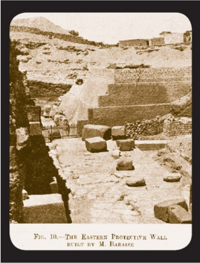
Figure 6.43. Selim Hassan published this photo in his own excavation report to show the “huge barrage-like walls” built in 1926 by Baraize to hold back the sand so that it did not reengulf the Sphinx. The massive constructions are shown in the upper half of the photo. Hassan and his team had the unenviable task of getting rid of these walls. Often it is more difficult to clear away modern structures than ancient ones! (From Excavations at Giza, 1936–1937, volume VIII )
