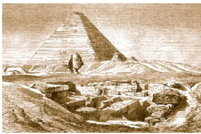
Figure 6.65. This nineteenth-century French engraving shows how Auguste Mariette excavated only the interior, but did not clear the exterior, of the Valley Temple at Giza during the years 1853–60. It is in the foreground, and at that time was called the Sphinx Temple, because the true Sphinx Temple had not yet been discovered. The head of the Sphinx is seen behind, and in the background is the Great Pyramid. ( Collection of Robert Temple )
