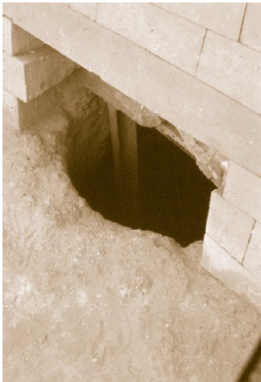
Figure 1.12. A close-up photo of the entrance to the rump tunnel. All the flat limestone blocks are modern reconstruction stones, not part of the original Sphinx. The way the bedrock has been cut away in a circular shape may here be seen clearly. The top of an interior modern steel support may also be seen. Behind the reconstruction blocks, a bit of the original Sphinx stone may be glimpsed above the hole. The rough workmanship and clumsy hacking evident here demonstrate that this is an intruded shaft from a late period that never formed part of the original intention of the Sphinx. It takes a thin person to squeeze inside. (Photo by Robert Temple)
