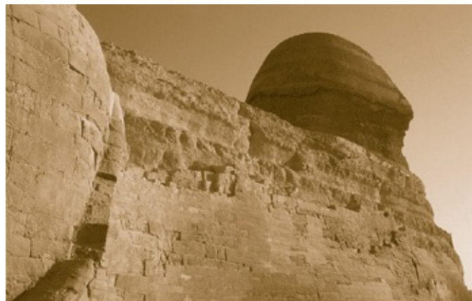
Figure 2.29. The filled-in waist on the right (southern) side of the Sphinx. The top half of the Sphinx's body seen in this photo is the original carved stone figure, deeply eroded in a series of horizontal stripes, whereas the bottom half is composed entirely of reconstruction blocks from different periods. These have had the effect of filling in the waist of the Sphinx, which was once narrow, thus disguising the doglike appearance and making the body appear to be more massive and leonine. At the left of the photo, the angle of the light on the tail enables us to see clearly that this portion of the tail at least is made entirely of blocks, and does not contain any carved stone core at all. The tail may therefore not be an original feature of the Sphinx but could have been added at a later period as part of a "lionizing" process. In any case, if there were an original tail, what we have now is largely or wholly a replacement, or "tail transplant." (Photo by Robert Temple)
