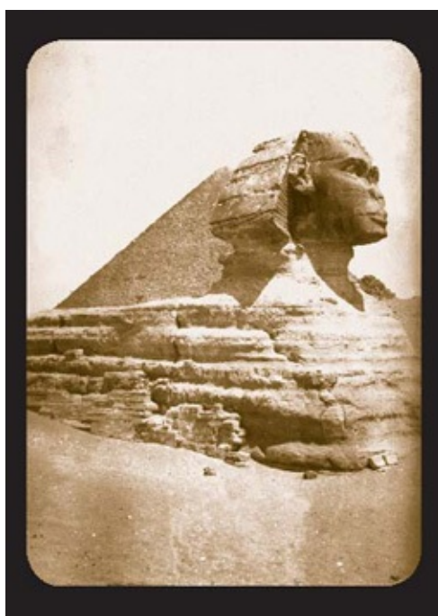
Figure 6.2. This photo, taken probably in the 1920s, shows the neck erosion of the Sphinx and the curiously pathetic attempt to fill holes in the right (southern) side of the Sphinx with stone blocks. They may have been covering an entrance into the Sphinx's body near one of the southern cupolas, or these blocks may merely be filling unsightly hollows. However, they were clearly intended to cover something, whether cosmetically or otherwise. This evidence should be taken into consideration when trying to decide whether the cupolas block an entrance to the body of the Sphinx. ( Collection of Robert Temple )
