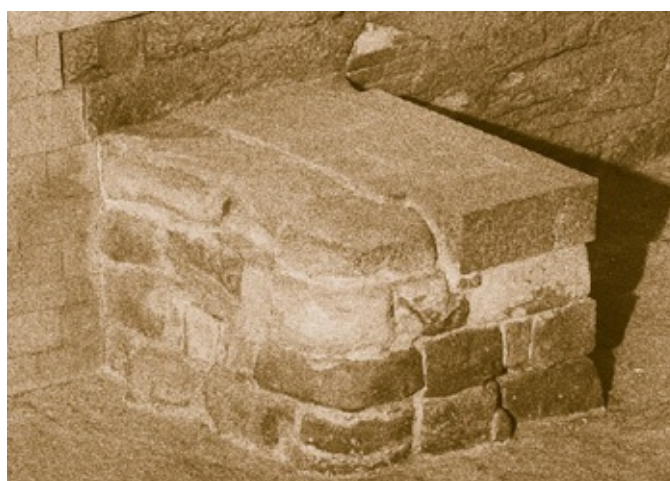
Figure 2.34. One of the four strange stone boxes protruding from the sides of the Sphinx at the base, presumed to have been constructed during the New Kingdom, perhaps to act as statue bases. This one is the smaller of the two that are on the south side of the Sphinx. The square stones on top at right are modern reconstruction stones, as are the small limestone pieces to the left of the box on the Sphinx's body. No one has any idea as to whether the four boxes sticking out of the sides of the Sphinx at the base might have been constructed to obscure an entrance into the body or to block an entrance to a shaft. Nor has any proper study of the four boxes ever been done, to my knowledge. None of the excavators ever paid much attention to them. It seems extraordinary to me that people just seem to accept the fact that there are four stone boxes protruding from the Sphinx. You would think that archaeologists would be rushing to examine them, study them meticulously, perhaps dismantle at least one and put it back together again (which would not be difficult), just in case there is something hidden inside. But no, nobody does anything. They just sit there and everybody ignores them. No one has even inserted any probes to see if they are hollow, as far as I know. Whoever said that human beings are curious? (Photo by Robert Temple)
