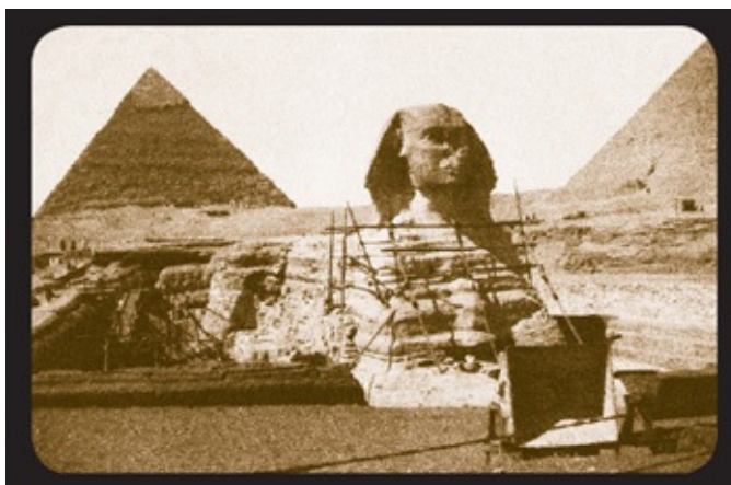
Figure 2.17. Here is the scaffolding platform used for smearing the modern cement onto the Sphinx's neck in 1936. At left, we see Selim Hassan's southern gangway descending from the Chephren Causeway into the Sphinx Pit on that side. ( Collection of
