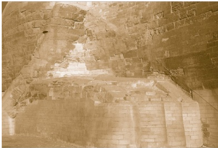
Figure 2.24. This photo of the Sphinx's right hind paw shows clearly how artificial it is and reveals the many layers of repair blocks. The pale small blocks are the new ones, made of freshly cut limestone and placed there in recent years to create a coherent tourist attraction that "looks right" from a distance. The protruding element behind the paw is the Sphinx's tail, which, as can be seen, consists now entirely of reconstruction blocks dating from different periods (the pale ones being the recent ones). To the right of the tail, and in the center of the photo above the paw, is the former giant crack in the Sphinx's body that can be seen so clearly in the 1921 photo shown in figure 1.31, before it was filled. In 1926, Baraize filled the crack by pouring in tons of cement and then covered over the cement with small limestone blocks (see at the top of this photo in the central portion). Below those, just above the paw, are a few courses of what appear to be older repair blocks, and to the left of them recent ones that are almost white, which have been stuffed in where some holes had begun to reappear since the 1920s. Those blocks to the left of the tail in this photo, which are large and worn, are thought to date from the Old Kingdom repairs. The small dark blocks at top right in this photo are probably Roman.
