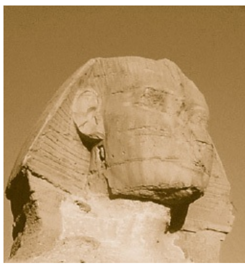
Figure 3.17. Here, the angle of the light enables us to see clearly the holes beneath the right ear of the Sphinx where the beard was affixed in later times. The modern concrete of the 1930s used as an extension of the side lappets of the nemes headdress is also clearly visible here, as is the way the bottoms of the stone portions of those lappets were chipped away to be level for the affixing of the modern concrete. (Photo by Robert Temple)
