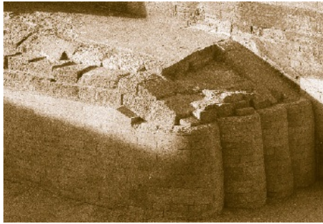
Figure 2.28. This rear right foot of the Sphinx is heavily restored by small, modern limestone blocks to make the monument presentable for tourists. (Photo by Robert Temple)
