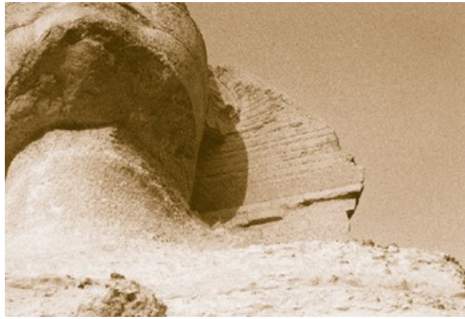
Figure 2.23. A close-up view of the left lappet of the headdress of the Sphinx. The bottom half of the lappet consists of a complex series of small restoration blocks, with a thin layer of slabs over them, followed by modern concrete up to the level of the original top half of the lappet. The effect from a distance is to make the lappet appear to be complete. (Photo by Robert Temple)
