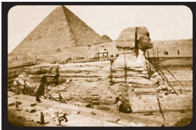
Figure 2.16. A snapshot taken by a tourist in 1936, during Selim Hassan's work on the Sphinx. The severely eroded stone of the uncovered rump is visible here from the side. As for the haunch area where the intruded shaft was, we can clearly see that Hassan erected special scaffolding to attend to that precise area. He must have found it necessary to add further filling and patching to Baraize's efforts of ten years before to fill in the broken-off haunch and smooth out the surface of the monument, restoring it to look like a single piece of sculpture again. The scaffolding erected in the front of the Sphinx has a platform used by masons to smear modern cement over the surface of the entire neck of the Sphinx. ( Collection of Robert Temple )
