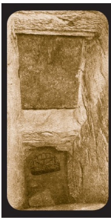
Figure 7.12. This photo shows very clearly the granite plug (top of photo) blocking the entrance to the Ascending Passage of the Great Pyramid from the Descending Passage. The plug is still there because entry to the Ascending Passage is from the forced passage made by al-Mamoun, which was tunneled through the limestone and went around it. This is plate LXVII on page 171 of John and Morton Edgar's The Great Pyramid Passages and Chambers , volume 1, Glasgow, 1910.
