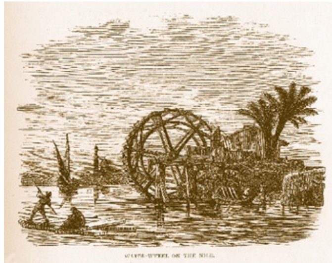
Figure 6.25. This is a noria water wheel, used for lifting quantities of water out of the Nile for irrigation purposes up until modern times. Although the noria did not yet exist in Old Kingdom times, as far as we know, it represents a successor to the shadouf system, which did exist then (see figures 6.26 and 6.27). At all times throughout history, the Egyptians have employed massive numbers of water-raising machines and shifted huge quantities of water. They were hydraulic engineers on a grand scale.
