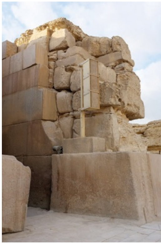
Plate 9. The northern entrance of the Valley Temple, showing the granite ashlars used to reface the older limestone blocks. (Photo: R. Schoch & C. Ulissey.)
