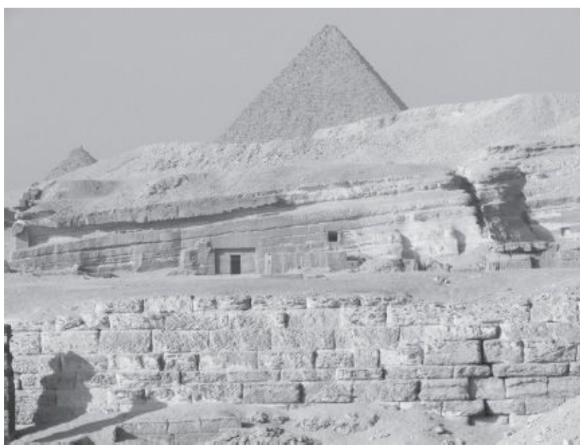
Fig. 7.18. Wind-induced weathering and erosion seen on Old Kingdom tombs of the Giza Plateau. (Photo courtesy of R. Schoch and C. Ulissey.)
