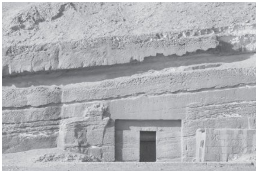
Fig. 7.19. Closer view of wind-induced weathering and erosion seen on Old Kingdom tombs of the Giza Plateau. (Photo courtesy of R. Schoch and C. Ulissey.)
