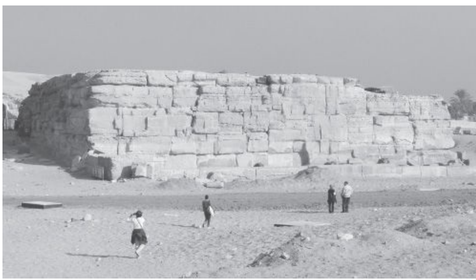
Fig. 7.16. The limestone core of the Valley Temple as seen from the south. (Photo courtesy of R. Schoch and C. Ulissey.)
