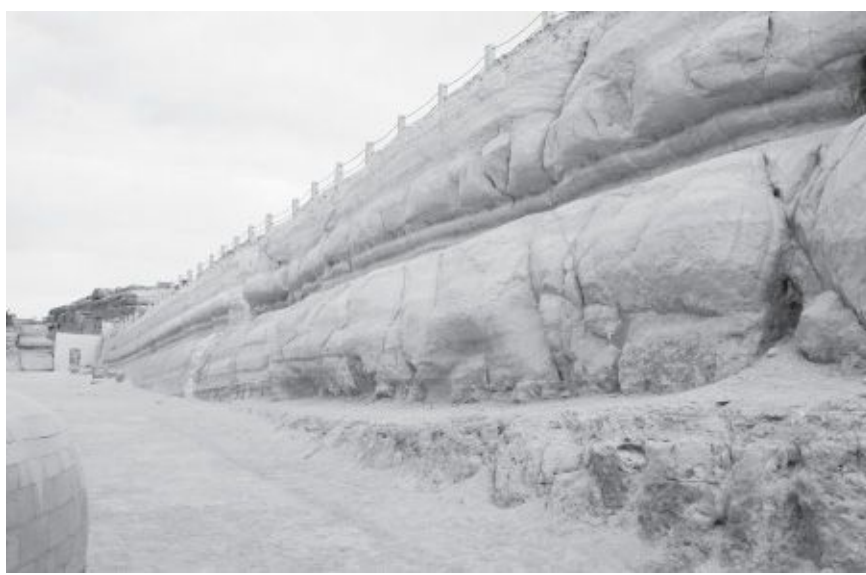
Fig. 7.22. Precipitation-induced (rain and water runoff) weathering and erosion on the southern wall of the Sphinx Enclosure. (Photo courtesy of R. Schoch and C. Ulissey.)
