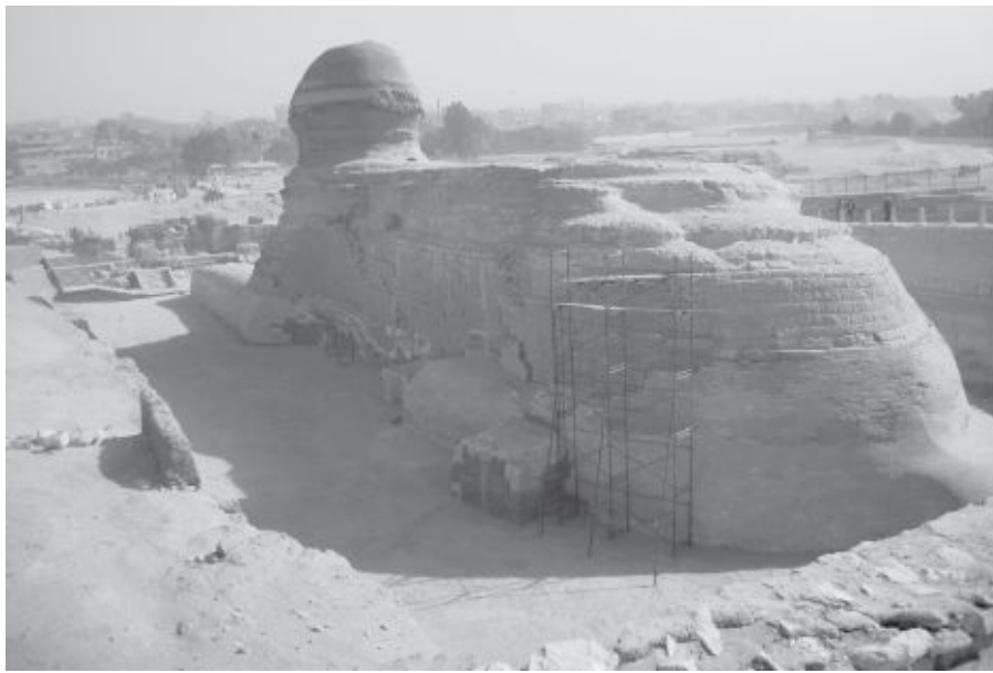
Fig. 7.9. View of the northern portion of the Sphinx Enclosure and the northern flank of the Great Sphinx showing various ancient and modern repairs to the Sphinx. (Photo courtesy of R. Schoch and C. Ulissey.)
