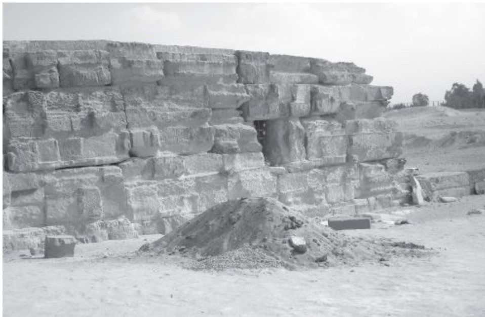
Fig. 7.15. The limestone core of the Valley Temple. (Photo courtesy of R. Schoch and C. Ulissey.)
