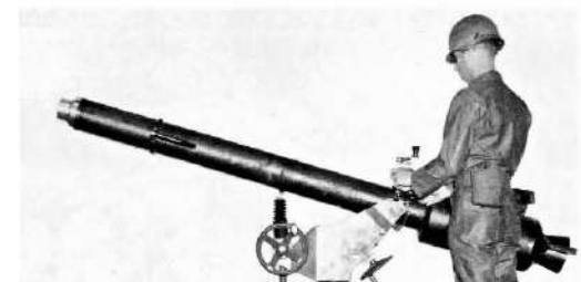
Unloaded M29 Davy Crockett (includes the M64 recoilless gun on a bracket mount, plus (1) the gun barrel seated M2 launching piston/spigot cylinder and (2) either of two fixed propellant charges/cartridges, M76 (or M94) "Zone I" or M77 "Zone II", seated in the M64's chamber).
