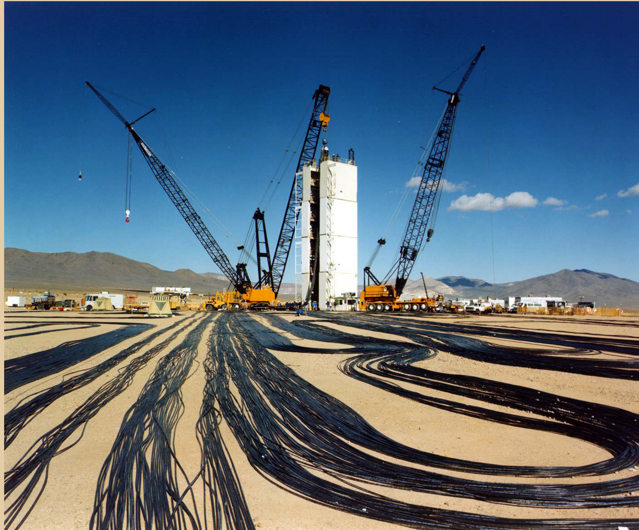
Preparations take place in Nevada for an underground nuclear test. The test site or box, the place the nuclear device will be detonated, lies 100s of feet below ground, below the base of the tower in the background.
