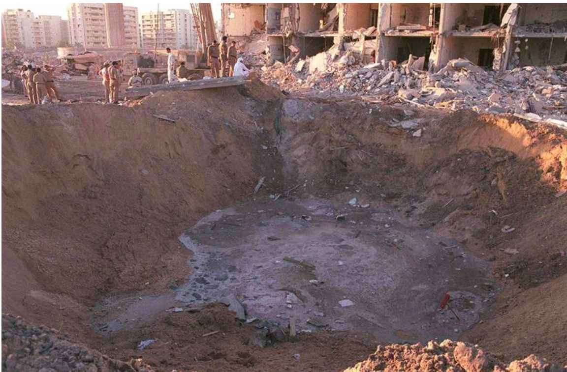
Crater left by the “truck-bomb” used in 1996 Khobar Towers bombing. The official U.S. military photograph.
