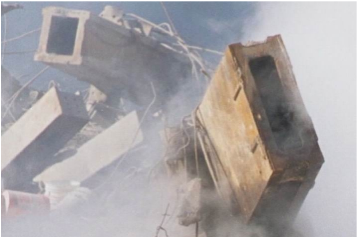
Some remaining perimeter- and core columns of the Twin Tower at “Ground Zero”.
