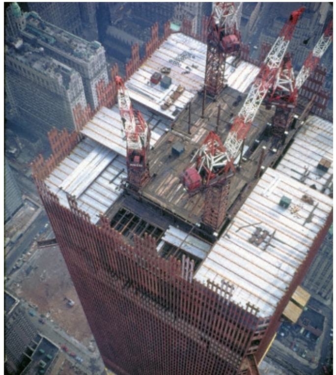
Above: steel perimeter columns of the WTC during its construction.
