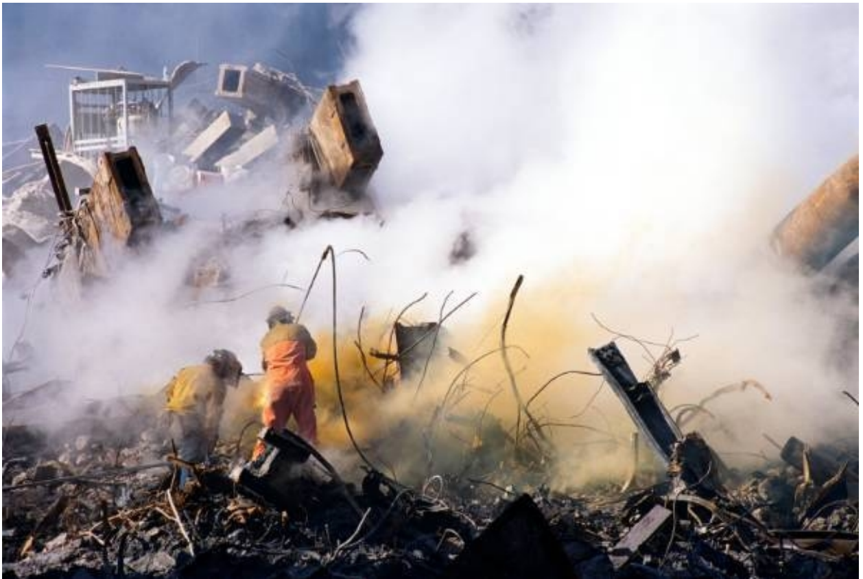
Above – remaining perimeter- (square) and core- (rectangular) columns of the Twin Towers at “ground zero” (amidst deadly radioactive vapors ascending from under the rubble).
