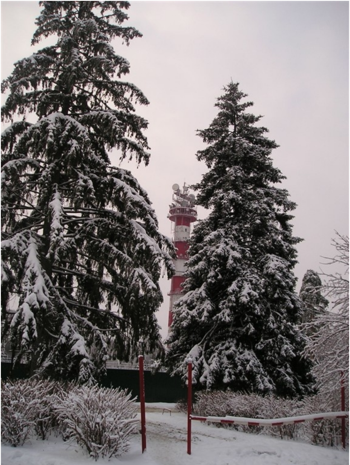
Above – a 120 meters tall TV-tower located in our village.
