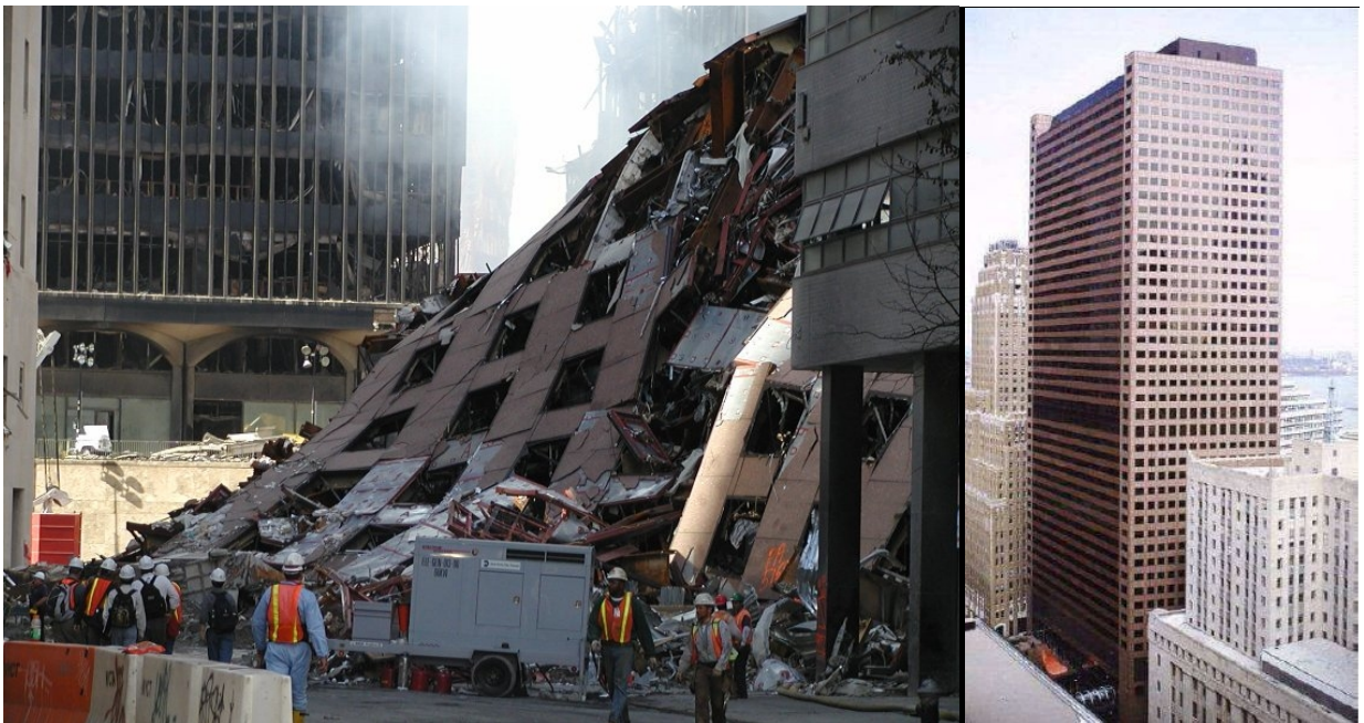
Above left – 5-stories high pile of debris left by the WTC-7 collapse. Above right – the 47-stories high WTC-7 building during its life time.
