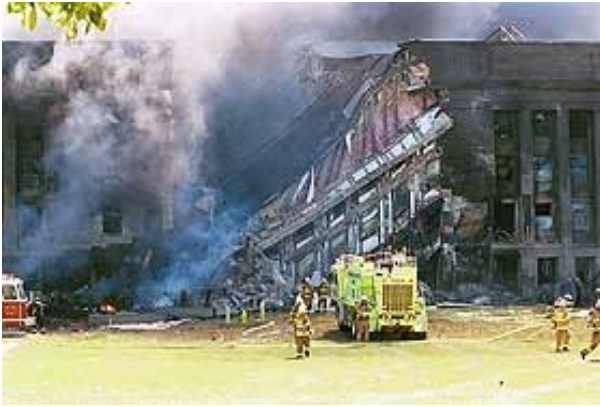
Pentagon's wall collapses 29 minutes after the attack.
