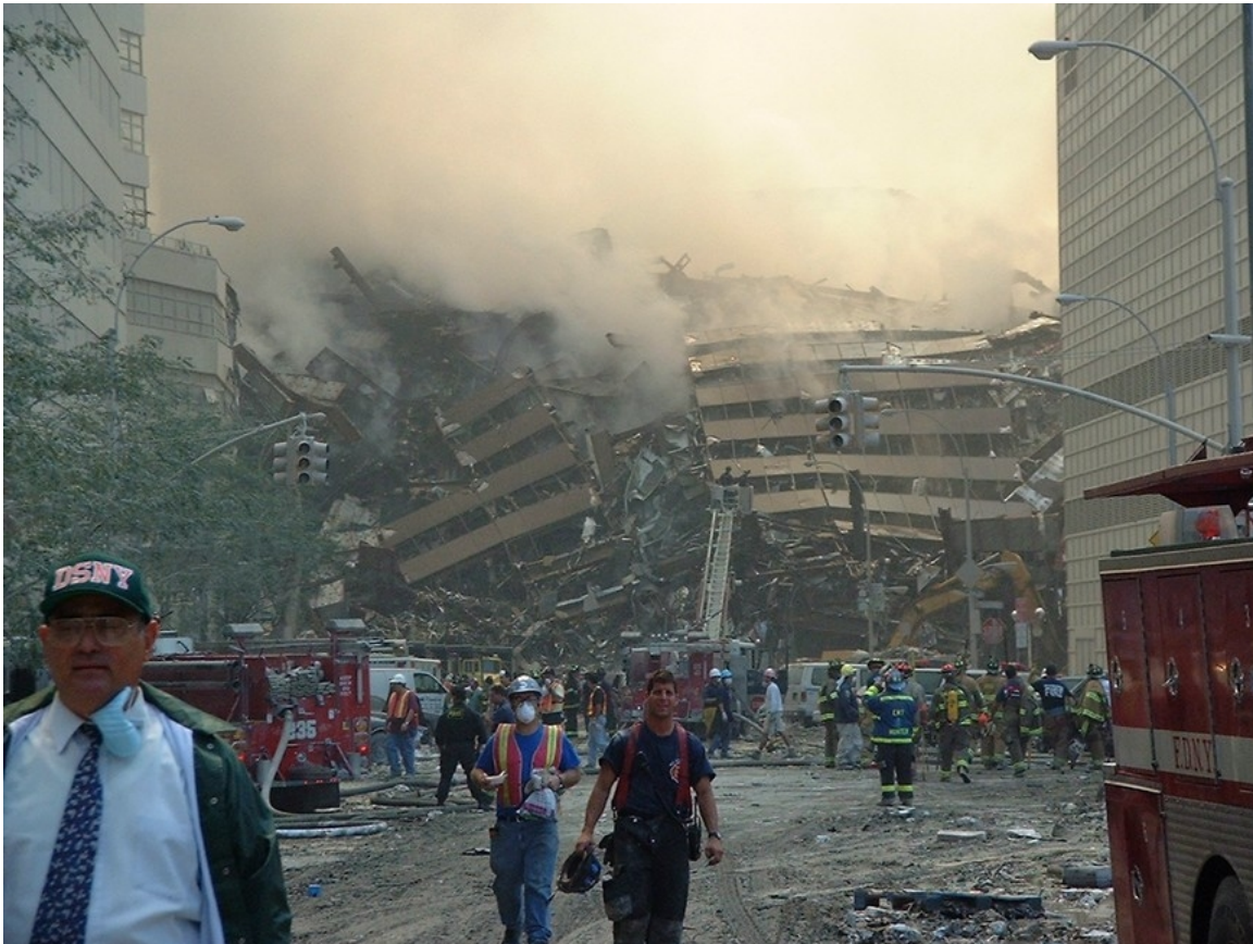
Above – the pile of the WTC-7 remains soon after its collapse.
