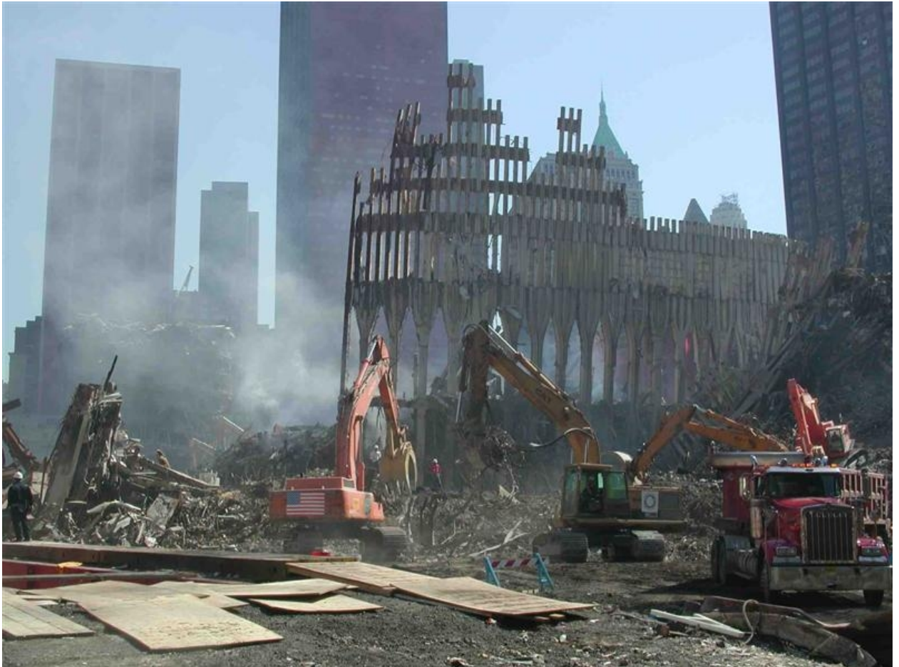
Perimeter columns of the South Tower that managed to survive pulverization.
