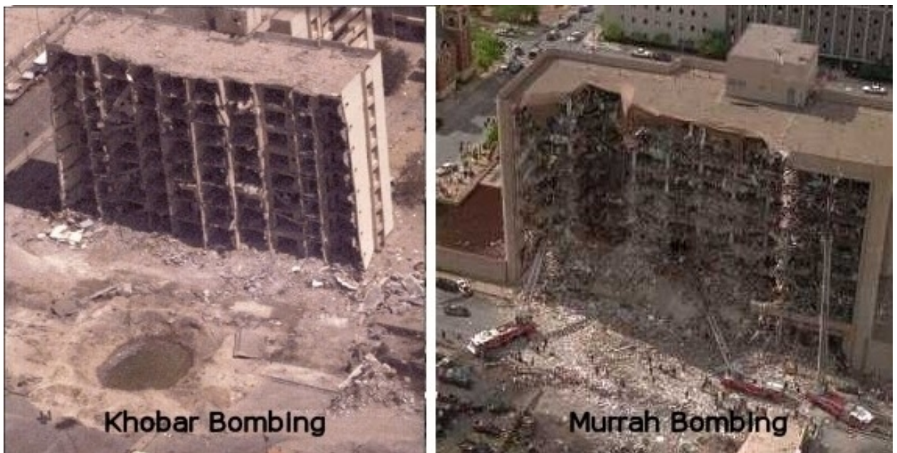
Comparison of the destruction caused by the 1995 Oklahoma bombing and the 1996 Khobar Towers bombing.
