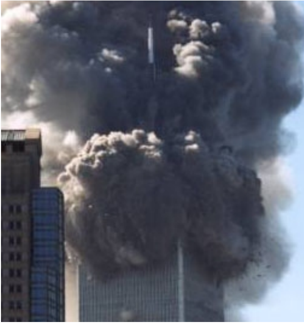
The top of the North Tower at the very beginning of its collapse.
