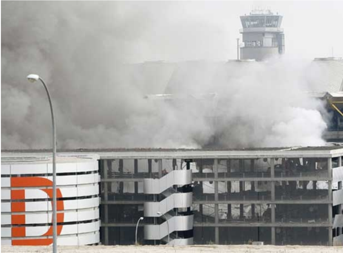
Barajas airport Terminal 4. Vapors ascending from the explosion area. It reminds one of those “unexplainable” vapors ascending from “Ground Zero” in Manhattan in 2001.
