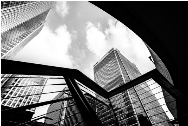
The former European Medicines Agency building at Canary Wharf, London, United Kingdom. Because of Brexit, in 2019 the EMA moved to Amsterdam.
