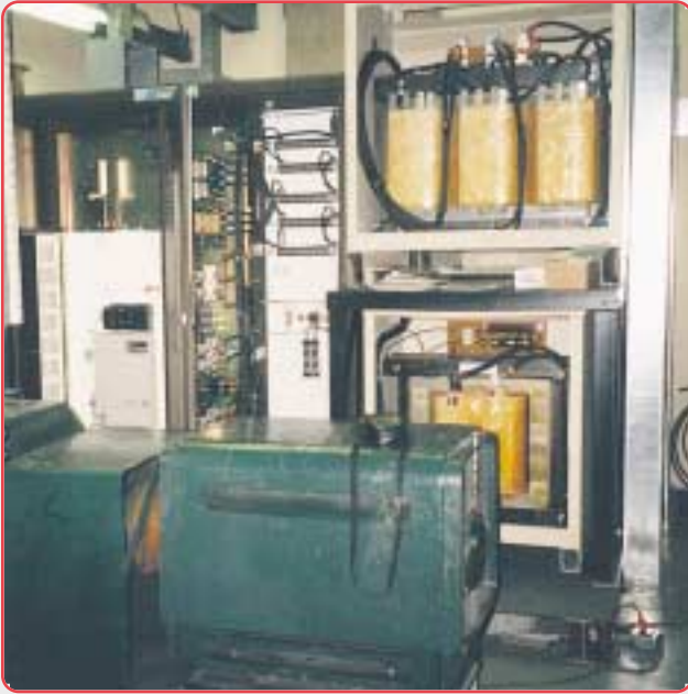
Motor generator room installation of the drive, choke and isolation transformer
