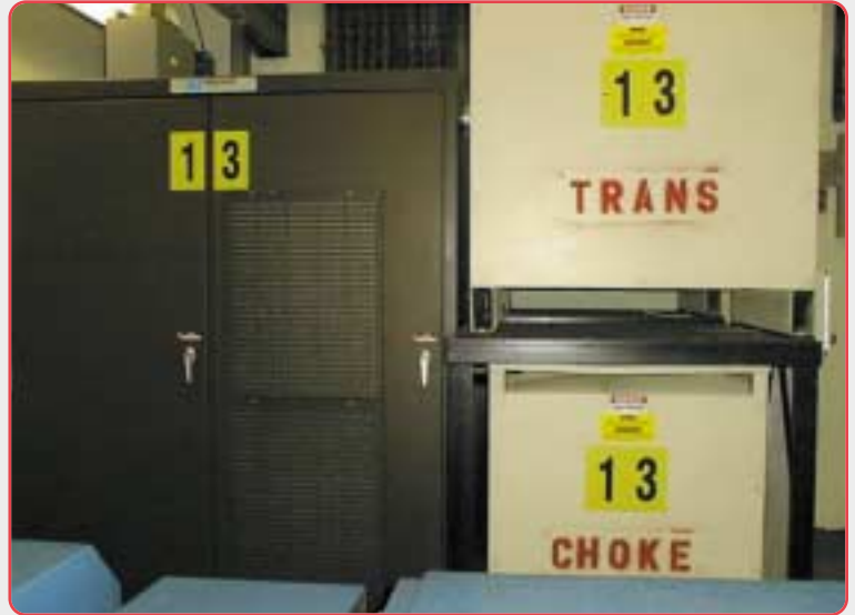
Motor generator room installation of the drive, choke and isolation transformer
