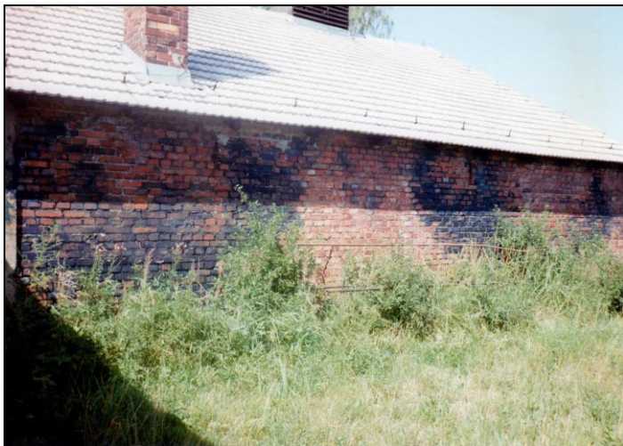
Illustration 22: Stained blue discoloration of the outer walls of the Zyklon-B-disinfestation wing of the hygiene Building 5b in Birkenau, Construction Section I (© Carlo Mattogno 1992).
