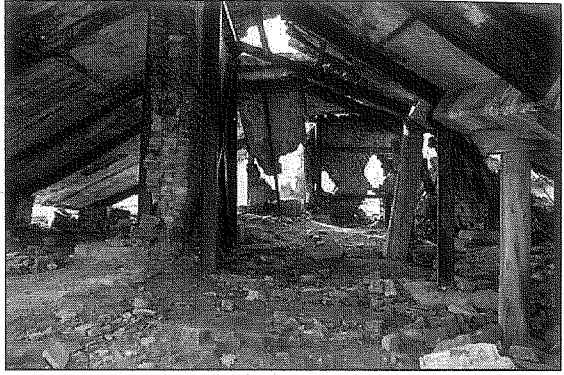
Illustration 14: Under the collapsed roof of the furnace hall of Kremas 2, Auschwitz-Birkenau.
