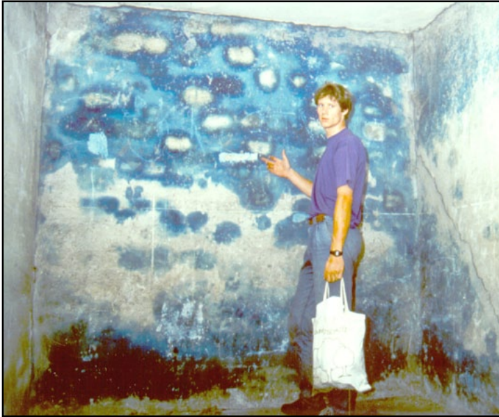
Photo 1: Interior wall of the disinfestation wing of Building 5a at Auschwitz-Birkenau
