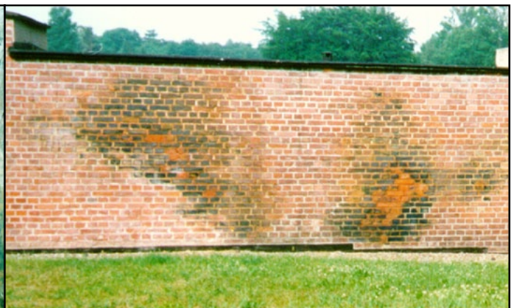
Photo 6: Exterior wall of the disinfestation facility at the Stutthof camp.
