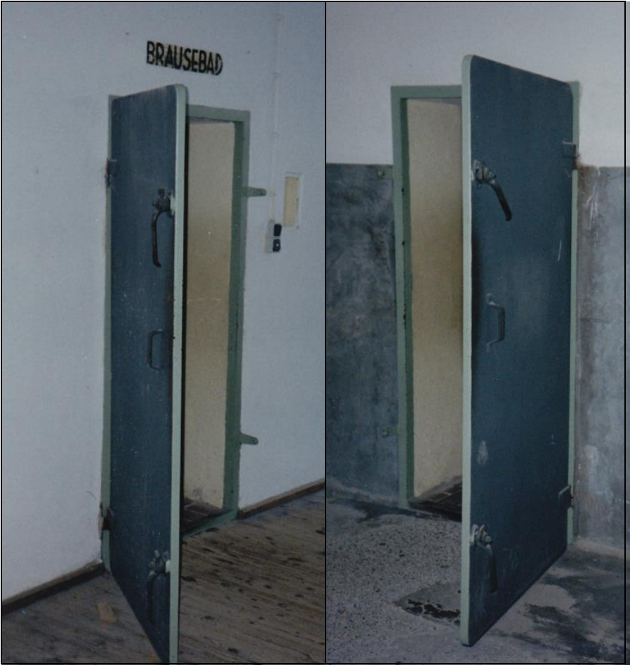
Photos 9 & 10: Entry- (left) and exit door of the alleged gas chamber at Dachau. December 1990. © Carlo Mattogno.
