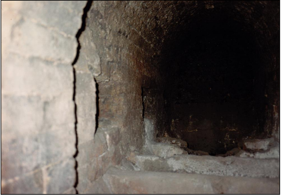
Photograph 145: as above, right-hand muffle, left-hand wall with rectangular openings to the center muffle.
