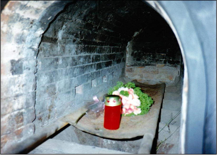
Photograph 52 & 53: Left-hand muffle. On the left muffle wall four holes for introducing combustion air can be seen. The grate bars are visible beneath the corpse-introduction stretcher.
