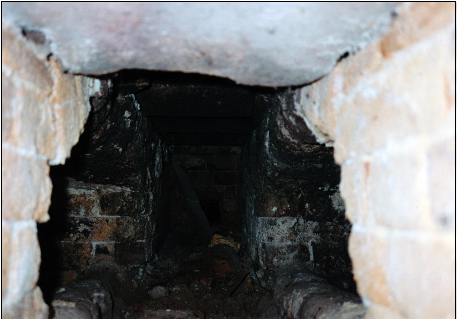
Photograph 156: as above, central muffle's ash chamber with the two lateral openings to the flue duct and a combustion-air-supply hole in the back.
