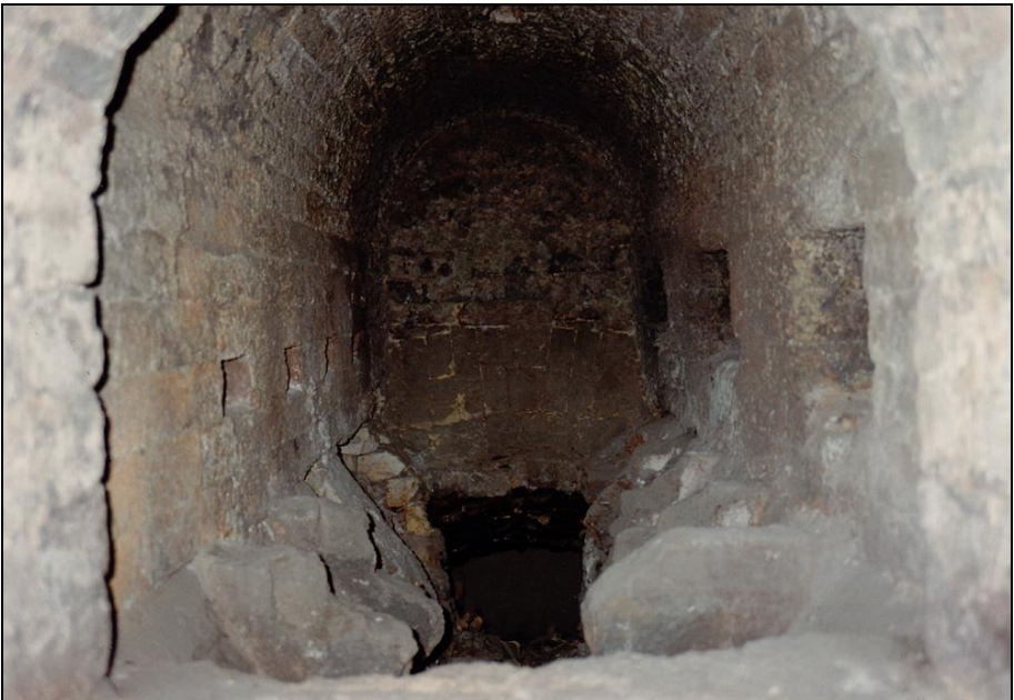
Photograph 140: Coke-fired triple-muffle furnace, left-hand muffle. Left wall: square openings of the combustion-air feed. Bottom: wall sloping into the ash chamber). Center bottom: opening to the gasifier. Right-hand wall: rectangular inter-muffle openings. The muffle-grate bars have been ripped out.
