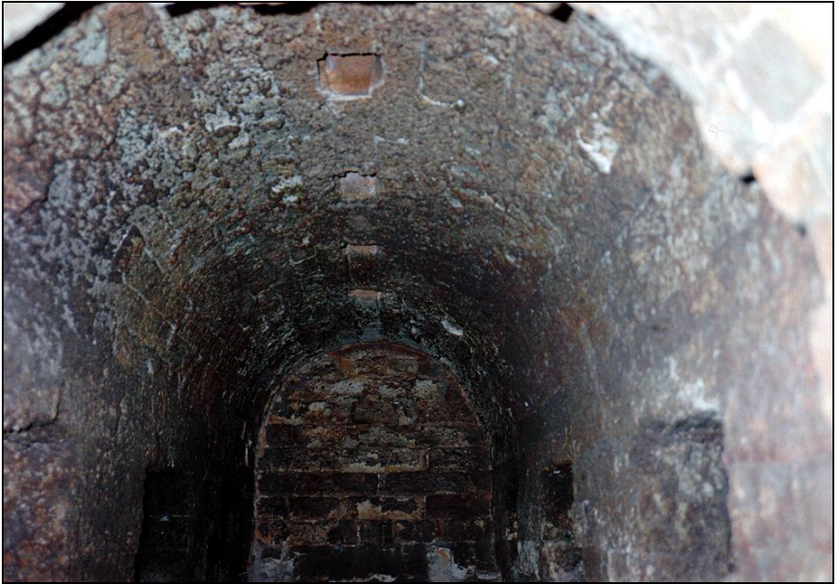
Photograph 137: as above, showing five of the rectangular inter-muffle openings, four square openings in the ceiling and one in the back wall for combustion-air supply.
