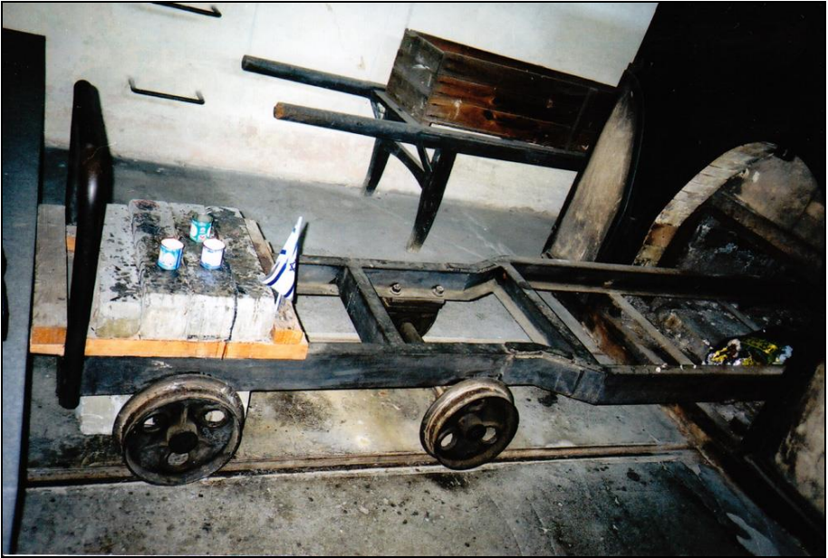
Photograph 361a: Left-hand furnace of the front pair, front view, with the corpse-introduction cart.
