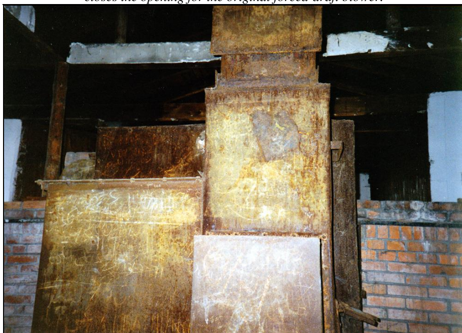
Photograph 48: Central part of the chimney.
