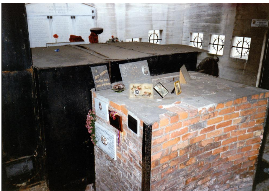
Photograph 35: Upper side of the furnace (from the right).
