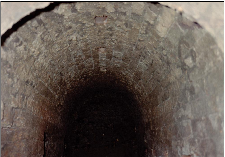
Photograph 146: as above, vaulted muffle ceiling with square openings for combustion-air supply.
