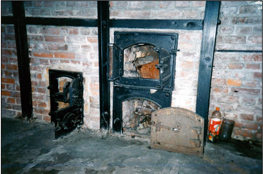
Photograph 276: Right-hand furnace. To the left: coke-loading door (center) and ash door (bottom) of the auxiliary gasifier. Center: double-leaf coke-loading door of the main gasifier with the ash-chamber door beneath.
