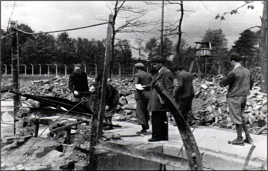
Photograph 225: as above; APMO, negative no. 21334/81.
