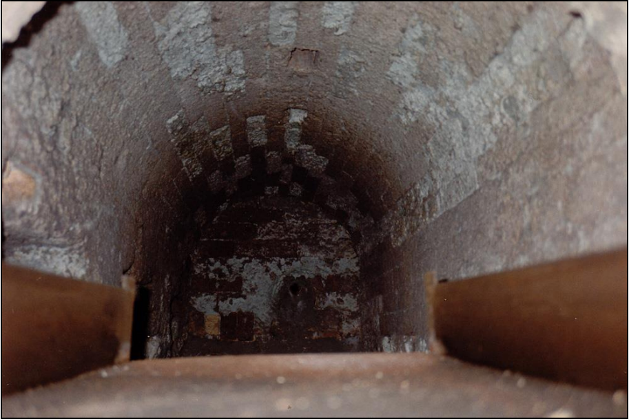
Photograph 139: as above; right-hand muffle. Foreground: the stretcher of the corpse-introduction cart. The opening of the naphtha burner can be seen in the wall in the background.
