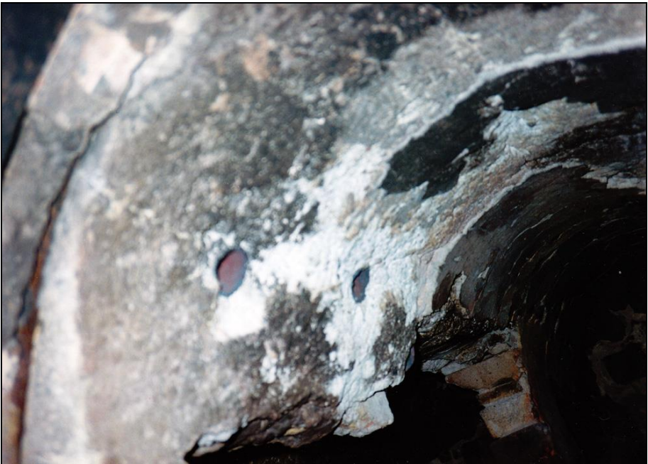
Photograph 42: Vaulted ceiling of the right-hand muffle; to the left: outlets of pipes connected to the blower.
