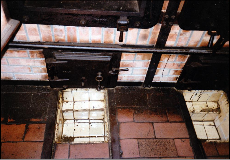
Photograph 155: TOPF coke-fired triple-muffle cremation furnace. Front-side service pits with the left and center muffle's ash doors.
