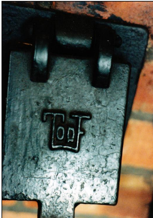
Photograph 154: combustion-air-channel door with the Topf insignia, close-up.
