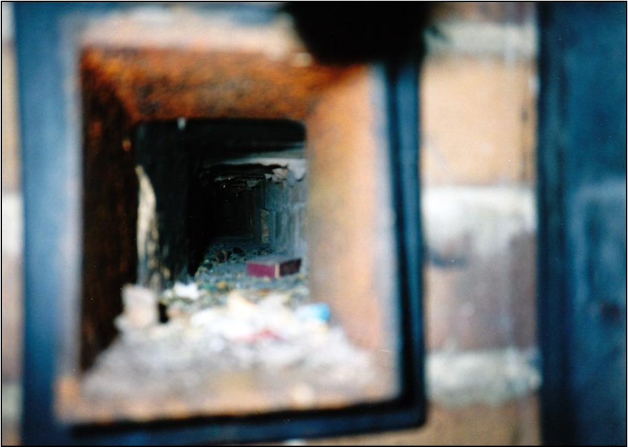
Photograph 57: Combustion-air channel of the left-hand muffle, closed with the door visible in the next photograph.
