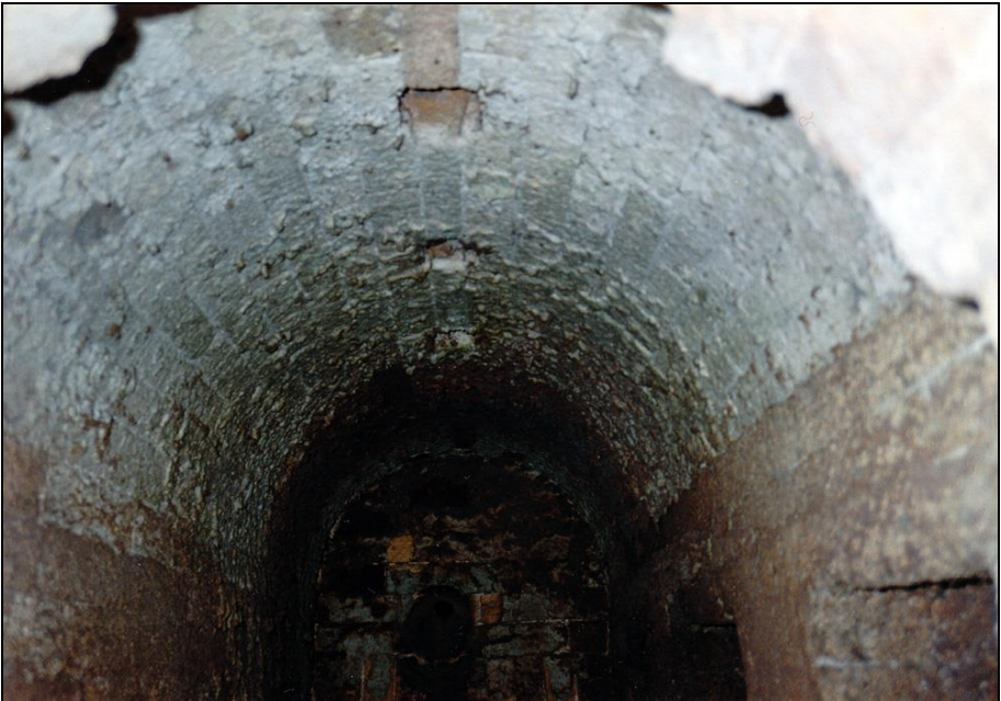
Photograph 132: as above; the apex of the vaulted ceiling sports four square openings which open into tubes supplying the muffle with combustion air.
