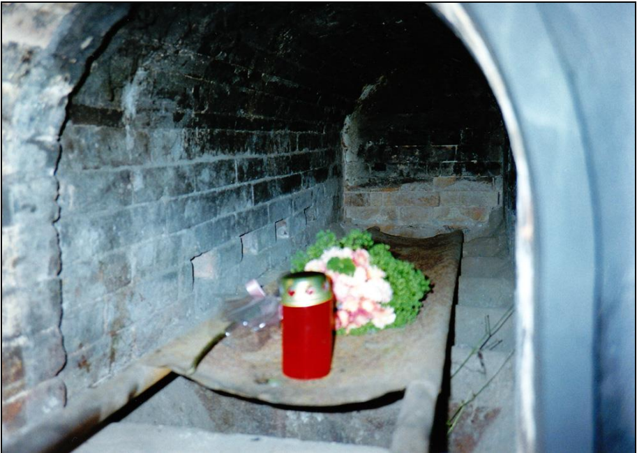
Photograph 52 & 53: Left-hand muffle. On the left muffle wall four holes for introducing combustion air can be seen. The grate bars are visible beneath the corpse-introduction stretcher.
