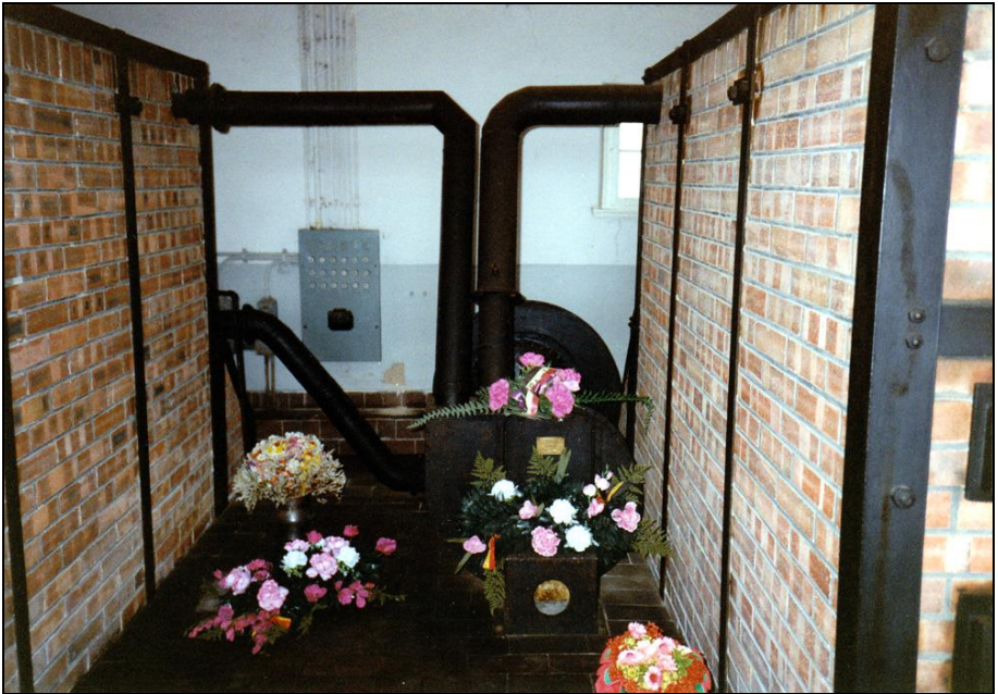
Photograph 188: Blowers located between the two furnaces.
