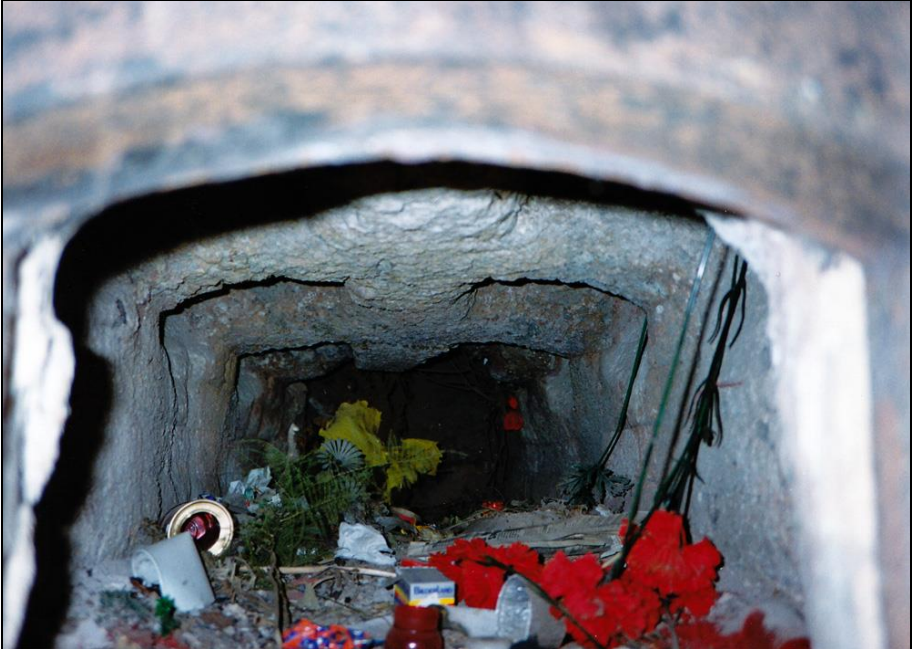
Photograph 243: ash chamber seen through the ash-chamber door.
