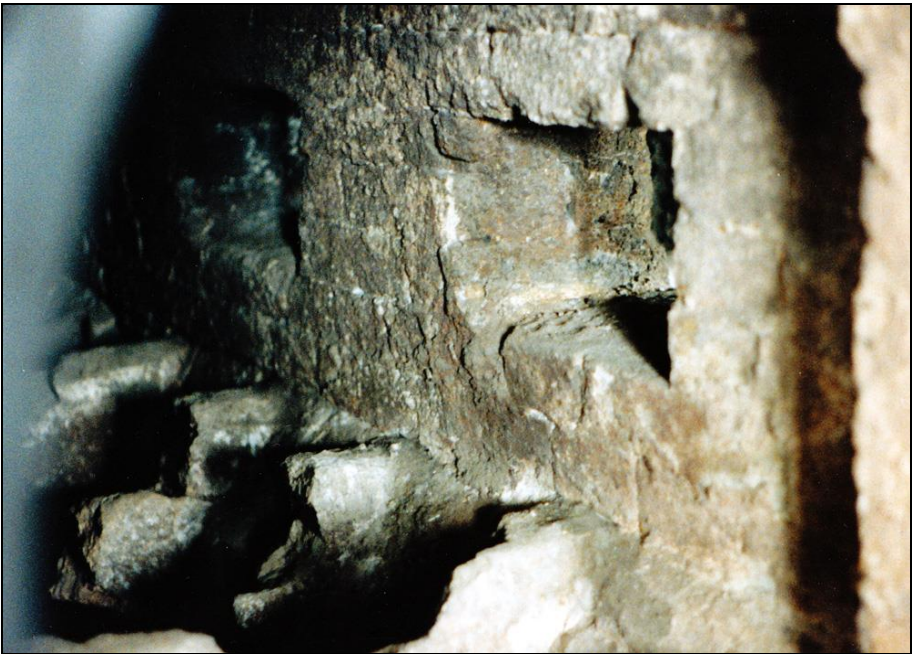
Photograph 144: as above, center muffle, right-hand wall with rectangular openings to the right-hand muffle.
