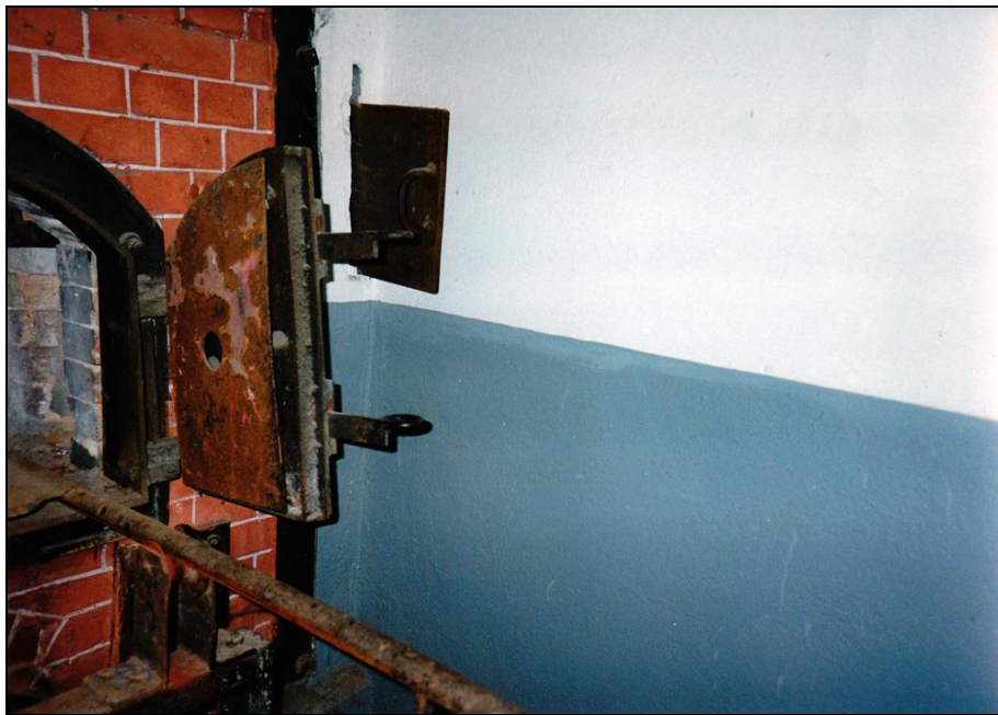
Photograph 238: as above, right-hand side; in the wall the chimney damper.
