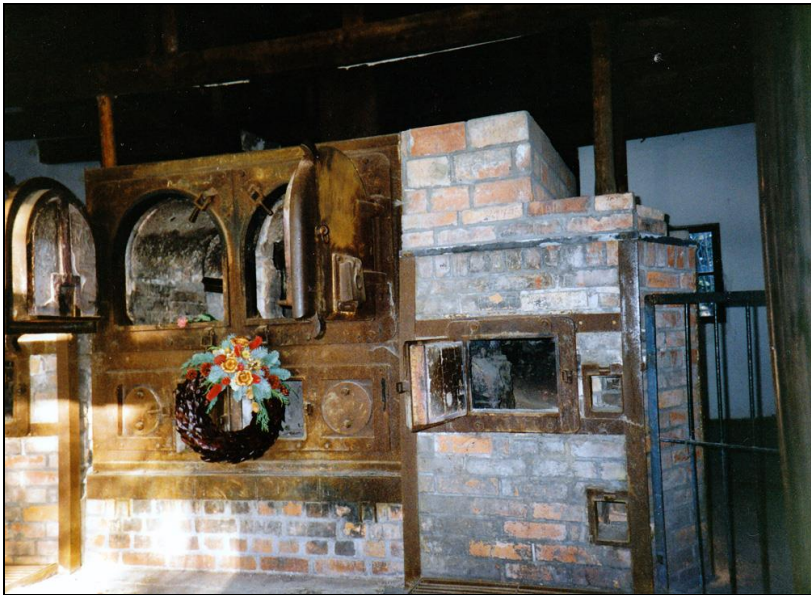
Photograph 38: Original furnace body with right-hand masonry gasifier.
