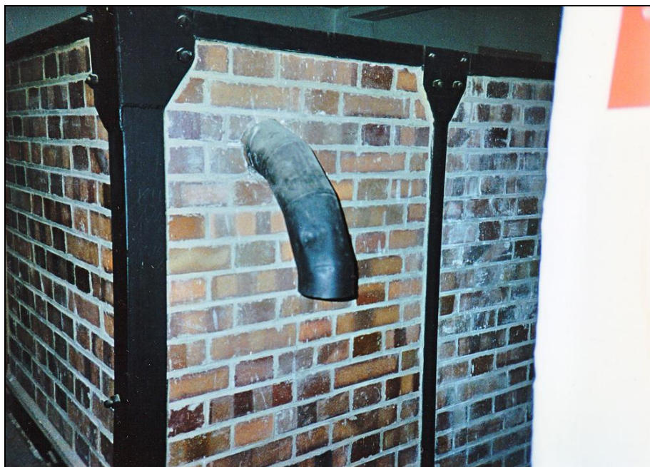
Photograph 76: Air pipe originally connected to a blower.
