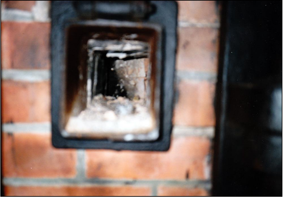
Photograph 151: as above, the muffle's combustion-air-supply channel.
