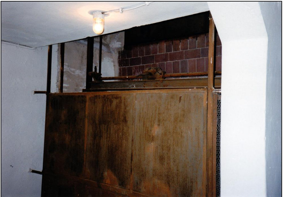
Photograph 213: as above, rear.
