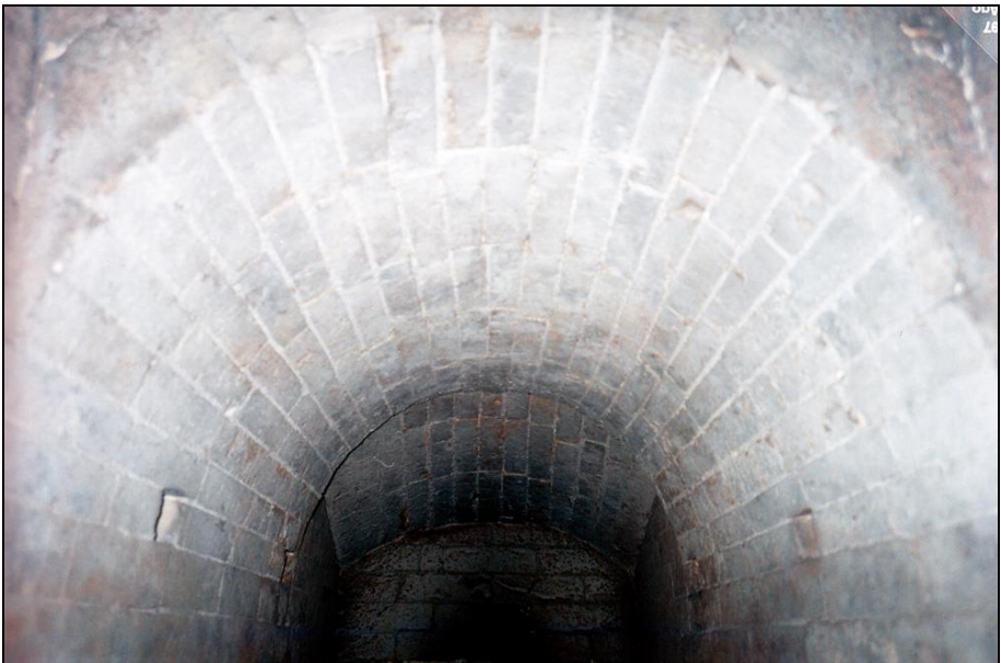
Photograph 297: Vaulted ceiling of the first muffle; in the side walls the openings of the combustion-air-supply channels can be seen.
