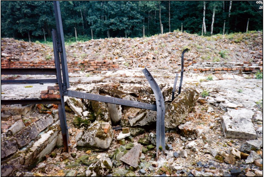
Photograph 230: as above; behind the iron frame: access ladder to the gasifier's service pit.
