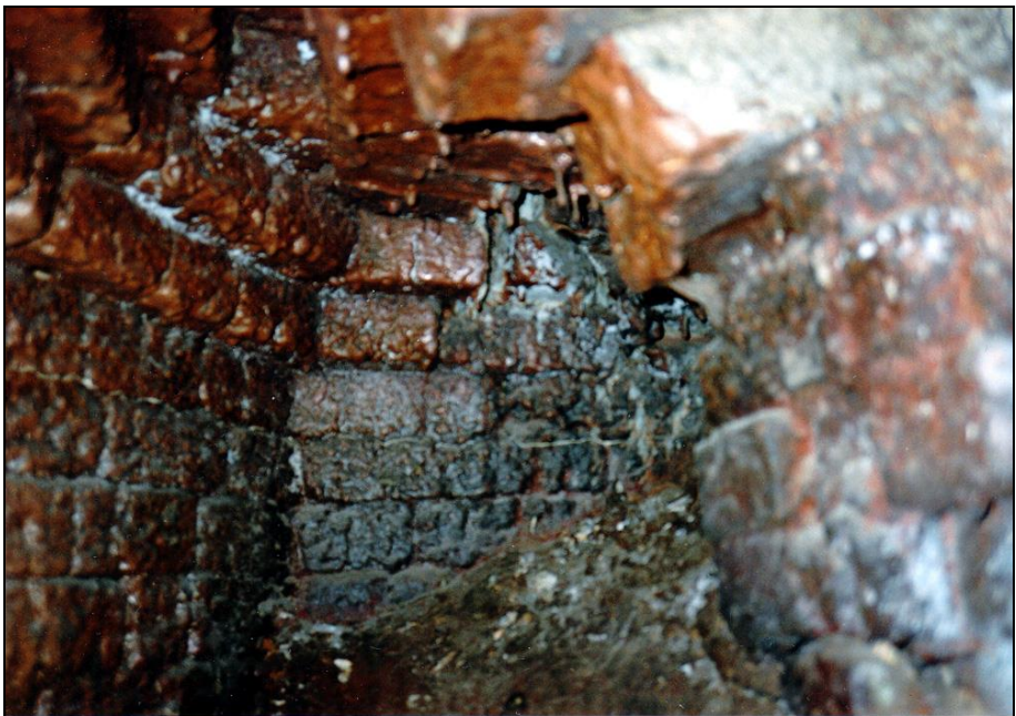
Photograph 5: Left-hand gasifier: Inside view, with the first opening connecting it to the left-hand muffle. The refractory brickwork shows evidence of fusion.
