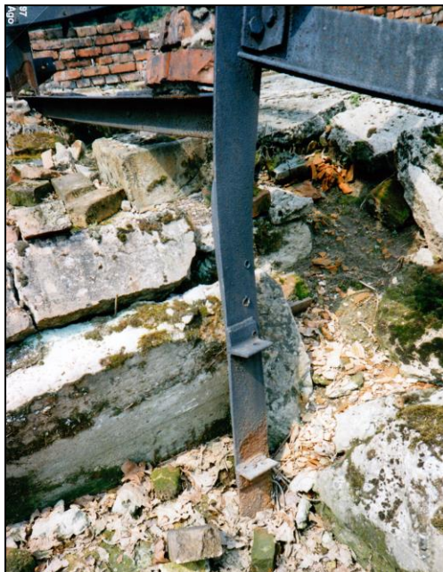
Photograph 231: as above. Detail of the northern gasifier's frame irons (direction south-north). The two brackets visible below were used for mounting the gasifier's hearth door.
