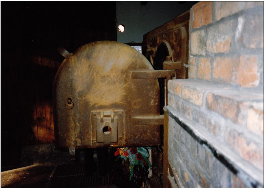
Photograph 44: Outside of left-hand muffle door.
