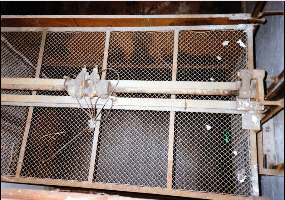
Photograph 215: as above; elevator cage viewed from the cremation hall above.
