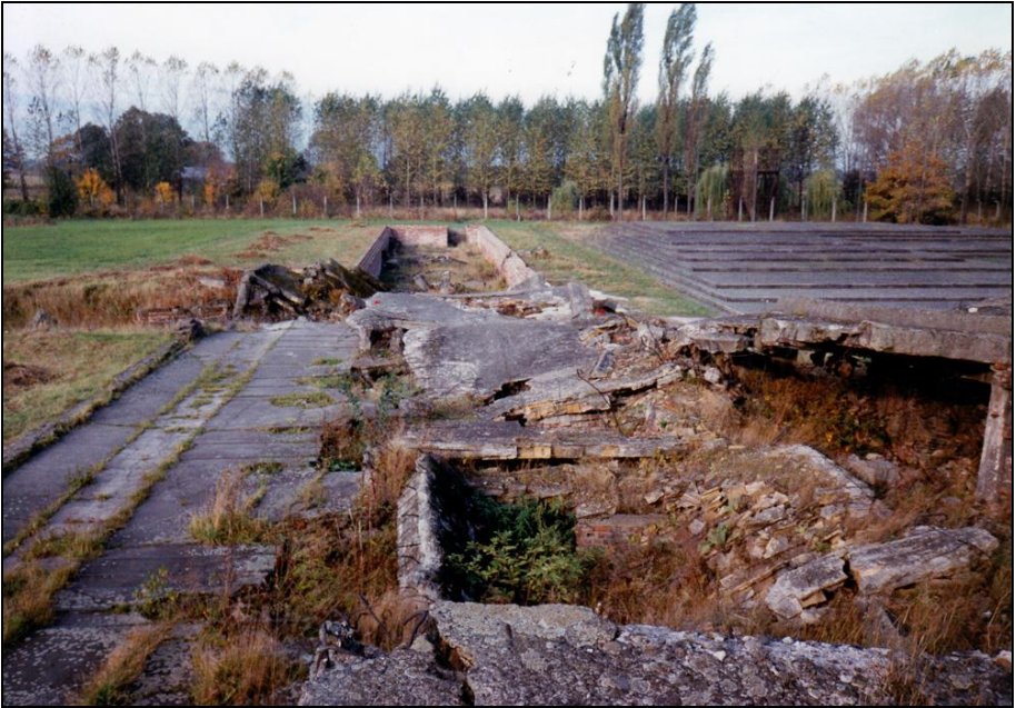
Photograph 221: as Photo 219; hole with the foundation of the chimney.
