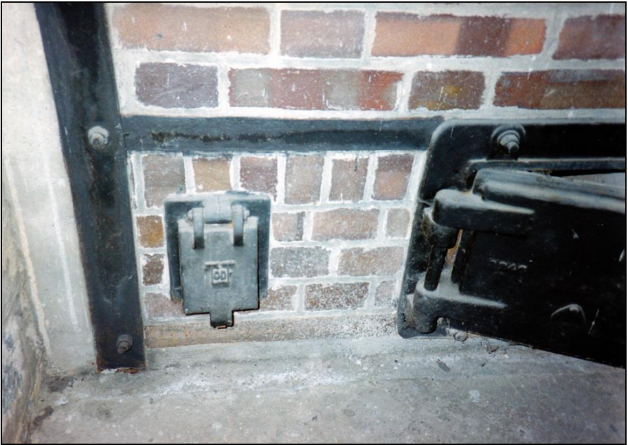
Photograph 81: as above; the left-hand combustion-air-intake door.
