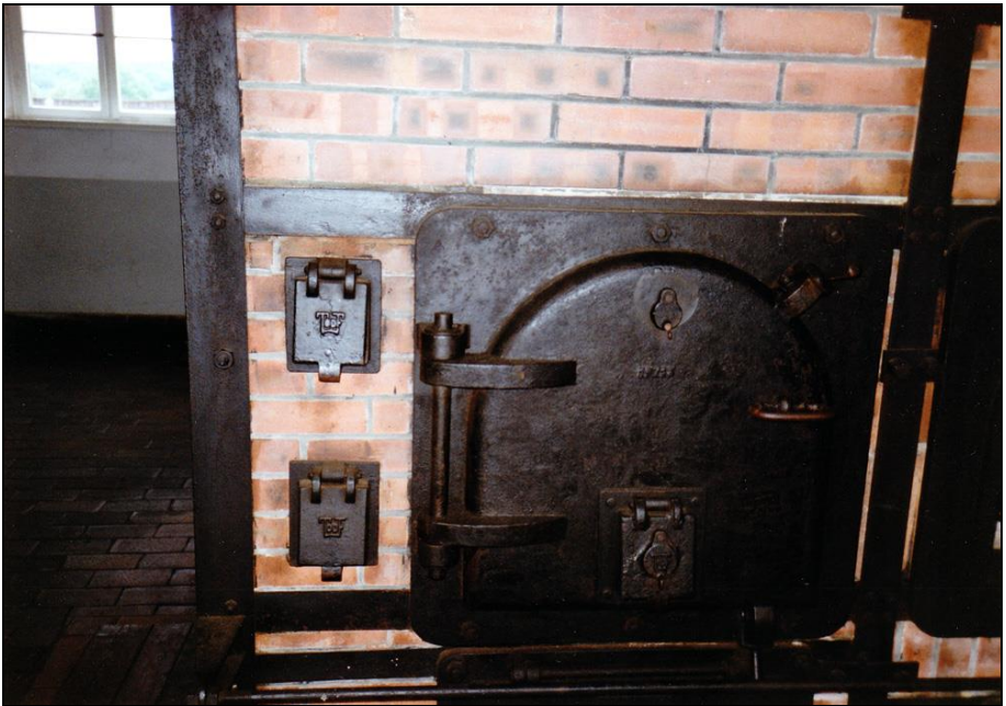
Photograph 150: as above, left-hand muffle. To the left of the large muffle door: doors closing the combustion-air channels of the muffle (top) and of the ash chamber (bottom).
