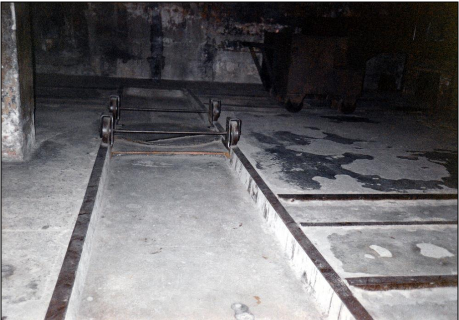
Photograph 105: Transverse rails and rotating platform (turntable).
