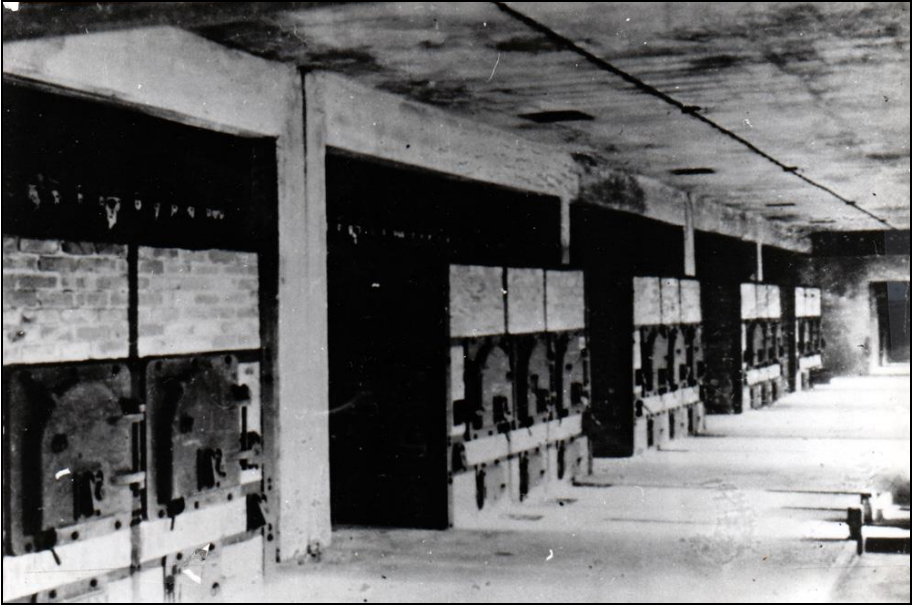
Photograph 115: SS photo of the TOPF coke-fired triple-muffle furnaces at Crematorium II at Birkenau. APMO, microfilm no. 290.
