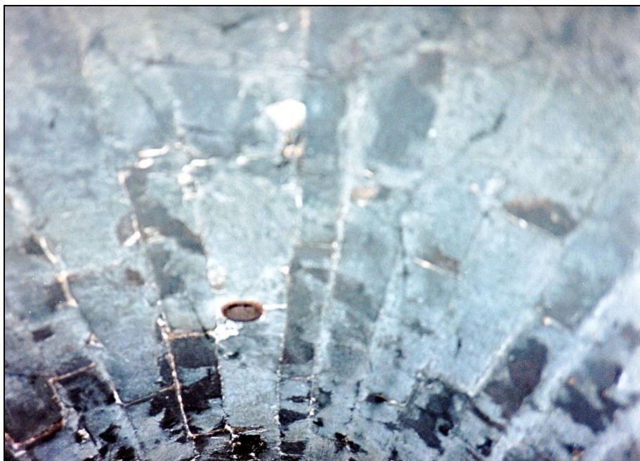
Photograph 60: Vaulted ceiling of the left-hand muffle; outlets of pipes connected to the blower.
