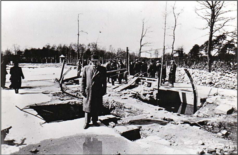
Photograph 222: Ruins of Crematorium V. Wrought-iron frame of the TOPF eight-muffle furnace and service pit. Polish photo of May 1945. APMO, negative no. 21334/141.
