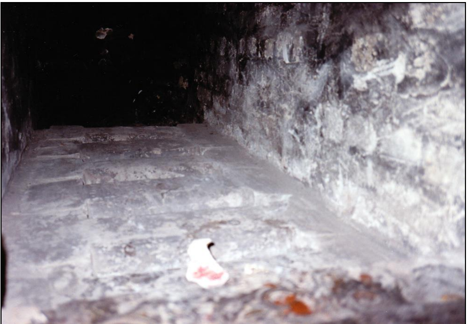
Photograph 93: Furnace no. 2: grate of the left-hand muffle.
