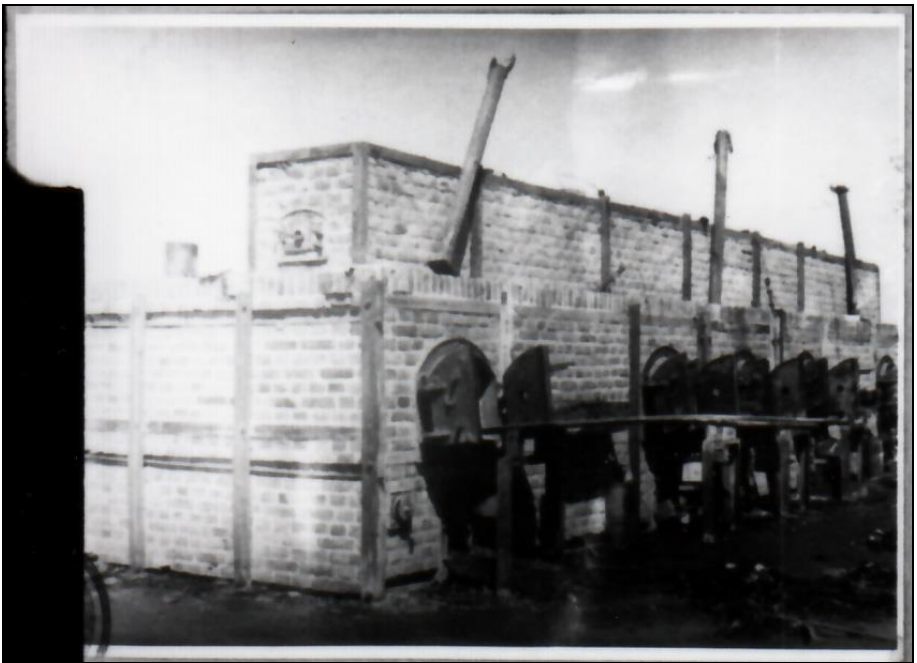
Photograph 286b: as above; the furnaces.
