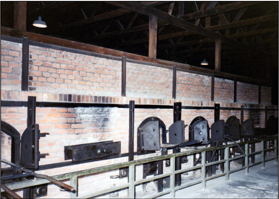
Photograph 287: Row of cremation furnaces with five muffles, front view.
