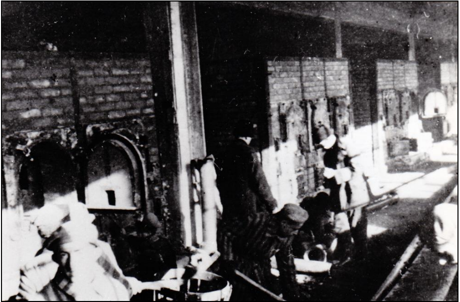
Photograph 113: SS photo of the TOPF coke-fired triple-muffle furnaces at Crematorium II at Birkenau. APMO, microfilm no. 290.
