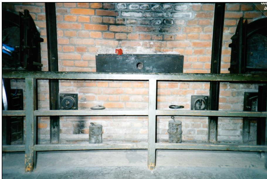
Photograph 289: as above; first recuperator.
