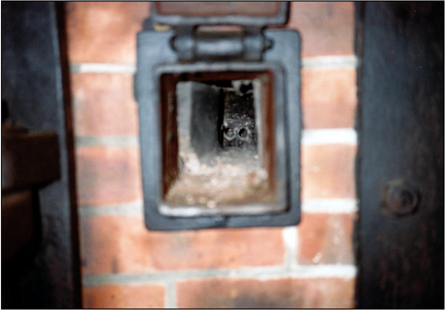
Photograph 149: as above, the muffle's combustion-air-supply channel.
