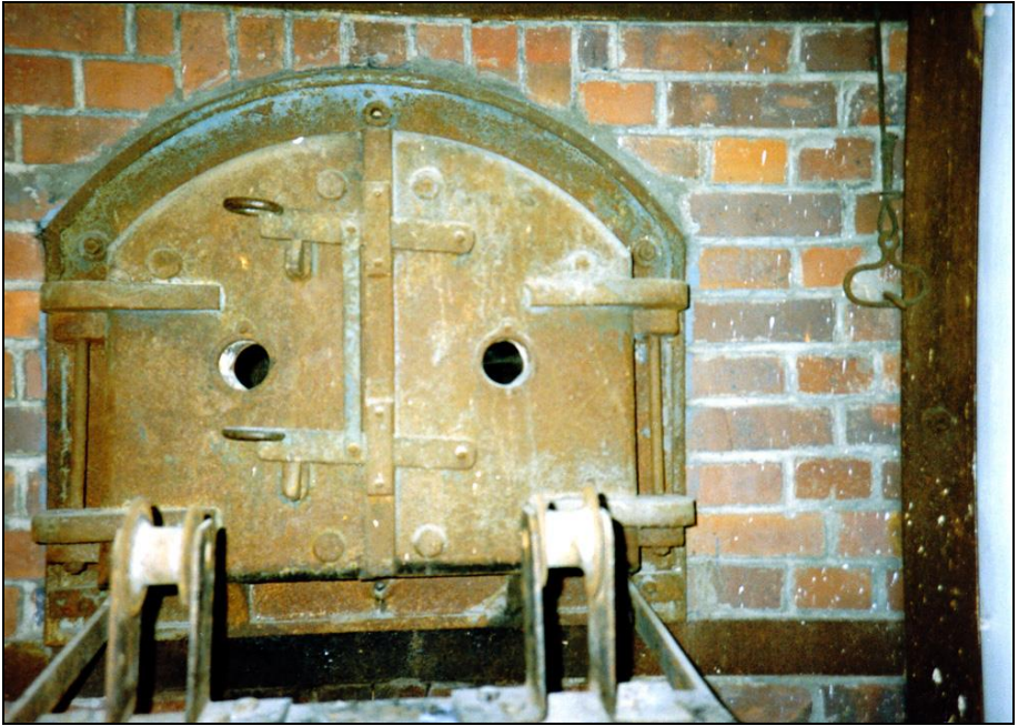
Photograph 252: as above, close-up of the muffle door.
