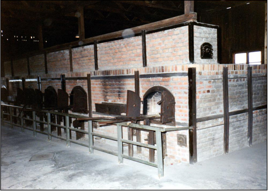
Photograph 309: Front view from the right-hand side. The brick structure at top contains the smoke duct, with an inspection door on the side.
