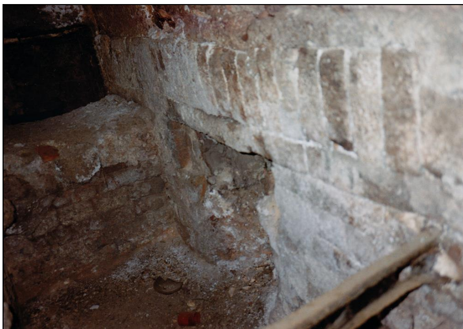
Photograph 27: Right-hand muffle: ash compartment with an opening connecting it to the gasifier.
