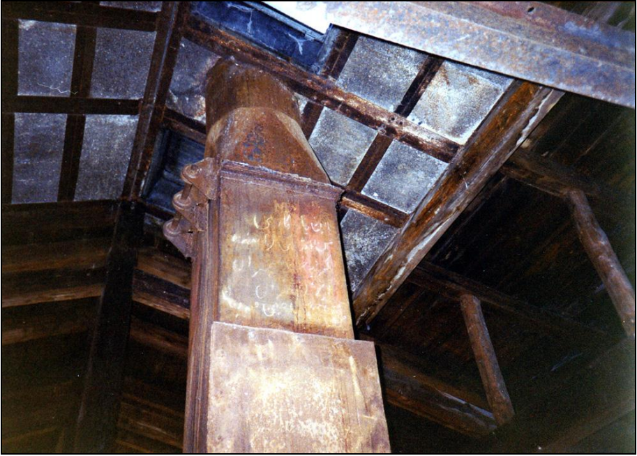
Photograph 49: Top part of the chimney.
