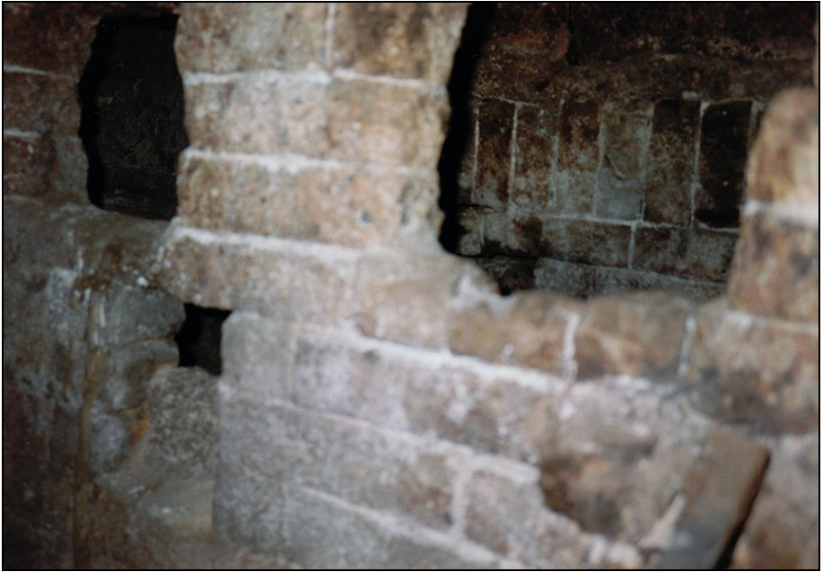
Photograph 20: Left-hand muffle: partition wall with inter-muffle openings.
