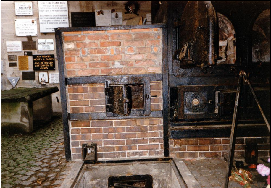
Photograph 4: The furnace's left-hand gasifier with coke-loading door and the gasifier's primary air-intake door (with the shutter missing).
