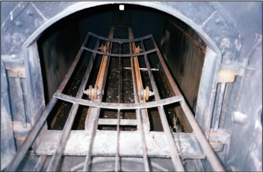
Photograph 334: Interior. The introduction stretcher moved with four metal rollers on two angle irons. The opening in the back wall housed the main burner. The refractory lining has been completely removed.
