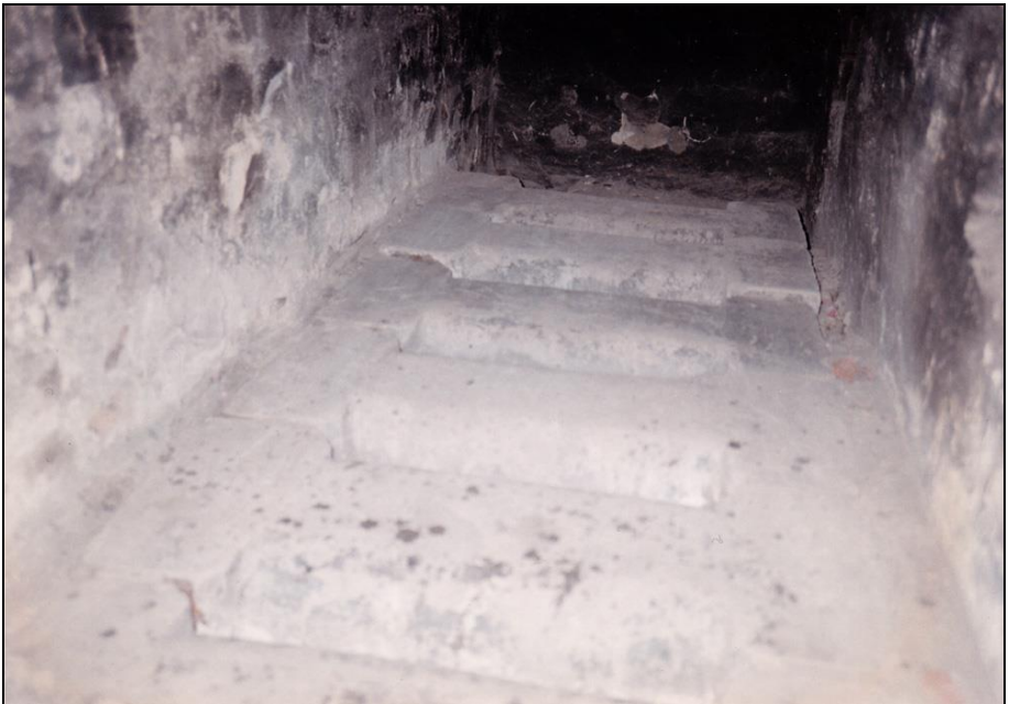
Photograph 95: as above; grate of the right-hand muffle.
