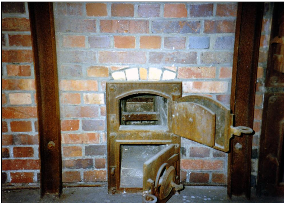
Photograph 260: First furnace, the auxiliary gasifier's service doors: loading door (top) and ash-chamber door (bottom).
