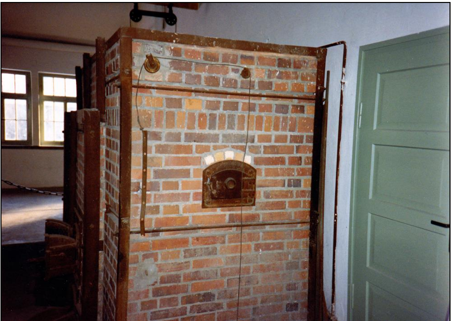
Photograph 259: Rear view of the first furnace; inspection door of the vertical smoke duct. Wire and pulleys for operating the smoke-duct damper, visible in Photo 258 on the floor at the bottom of the furnace.
