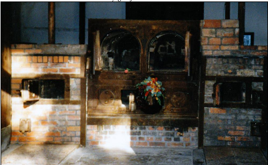
Photograph 36 (top) and 36a (bottom): Original furnace body of coated sheet metal with masonry gasifiers added to its sides.
