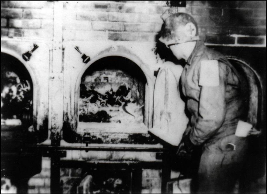
Photograph 206: A U.S. soldier in front of the central muffle of the TOPF coke- or naphtha-fired triple-muffle cremation furnace. U.S. Army photo of 1945.
