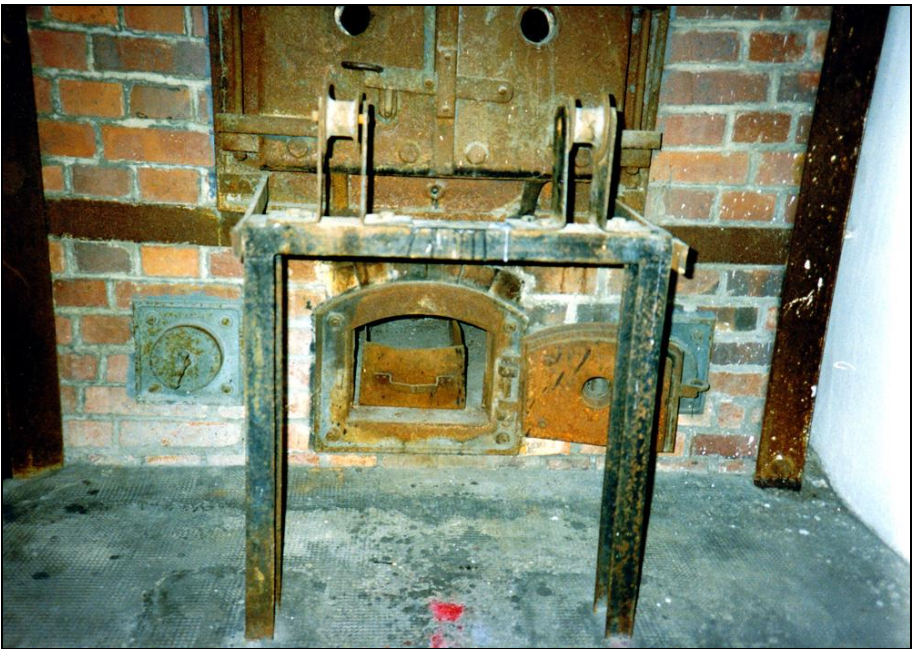
Photograph 251: as above, ash-chamber door and ash receptacle in the ash chamber; to either side: combustion-air inlets; foreground: metal stand with rollers for the corpse-introduction stretcher.
