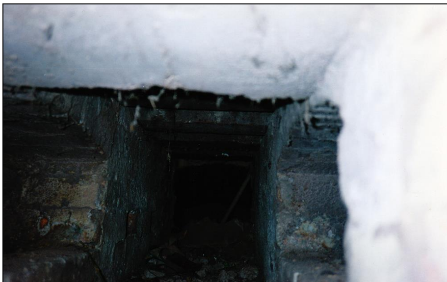
Photograph 72: Ash chamber of the left-hand muffle; at the top the bars of the muffle grate. On the left in the rear part of the wall are two small square openings of a combustion-air intake connected to a channel which opens on the left side of the furnace (see Photos 73f.). In front of those openings is the large opening of the flue-gas outlet; to the right the large opening connects to the ash receptacle of the right-hand muffle.
