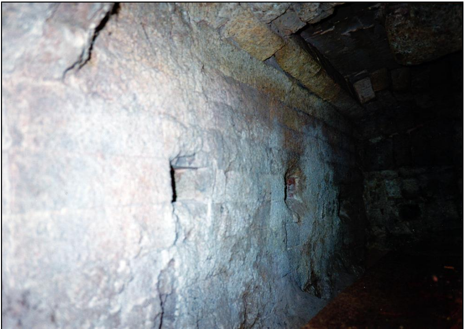
Photograph 241; as above, close-up of combustion-air-supply holes.
