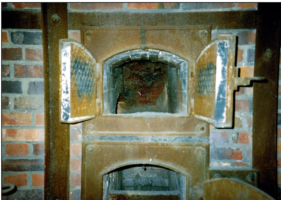
Photograph 261: Coke-loading door of the main gasifier.
