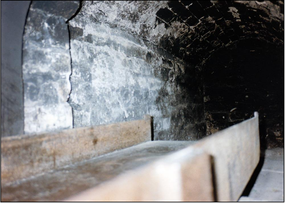
Photograph 92: Furnace no. 1: inside of a muffle. The masonry was artificially blackened.
