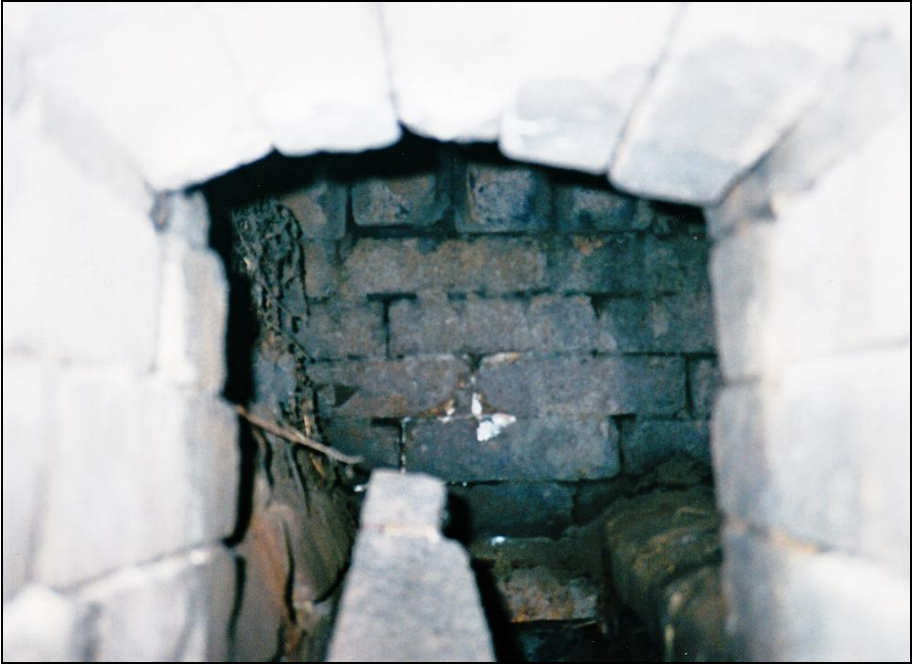
Photograph 281: as above. View into the auxiliary gasifier. Background: the wall of the muffle's ash chamber. Foreground: the end of an iron bar from the auxiliary hearth grate.
