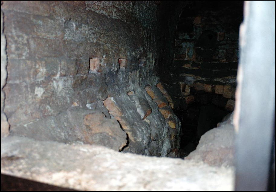
Photograph 131: as above; in the left-hand wall four openings of combustion-air channels are visible; below this the remnants of the muffle-grate bars and the walls slanted toward the ash chamber; in the back at the bottom is the opening to the gasifier.
