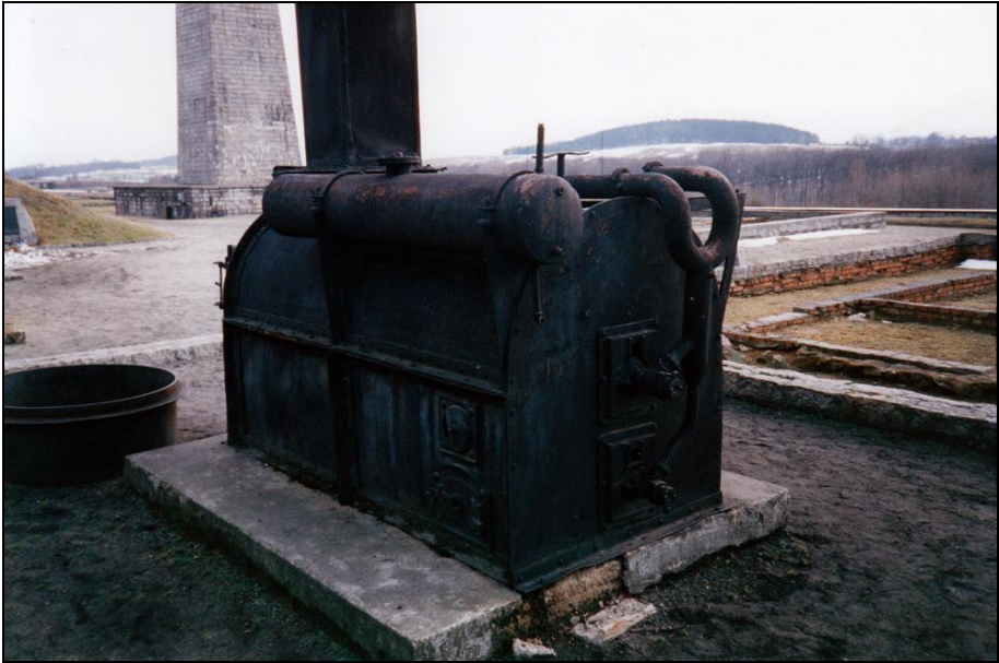
Photograph 333a: rear view. Left-hand side: naphtha tank; below it: combustion-air inlet and access door; right-hand side: combustion-air pipes; rear end: main (top) and auxiliary burner (bottom).
