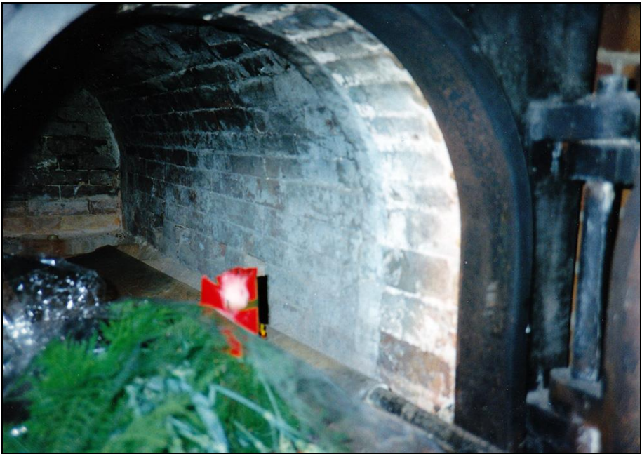
Photograph 55: Right-hand muffle. On the right muffle wall four holes for introducing combustion air can be seen..
