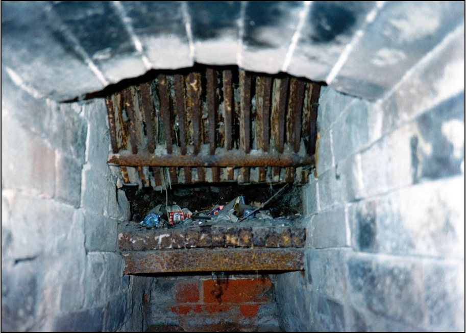
Photograph 246: gasifier grate.
