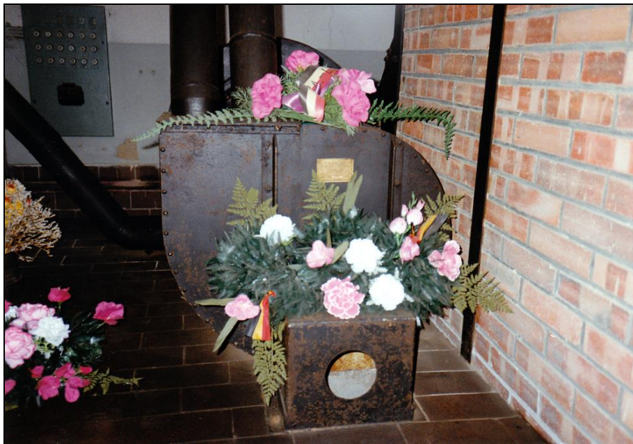
Photograph 189: The furnaces' combustion-air blower, front view; the left tube feeds the furnace heated with either coke or naphtha, the right tube the coke-fired one (see Photo 188).
