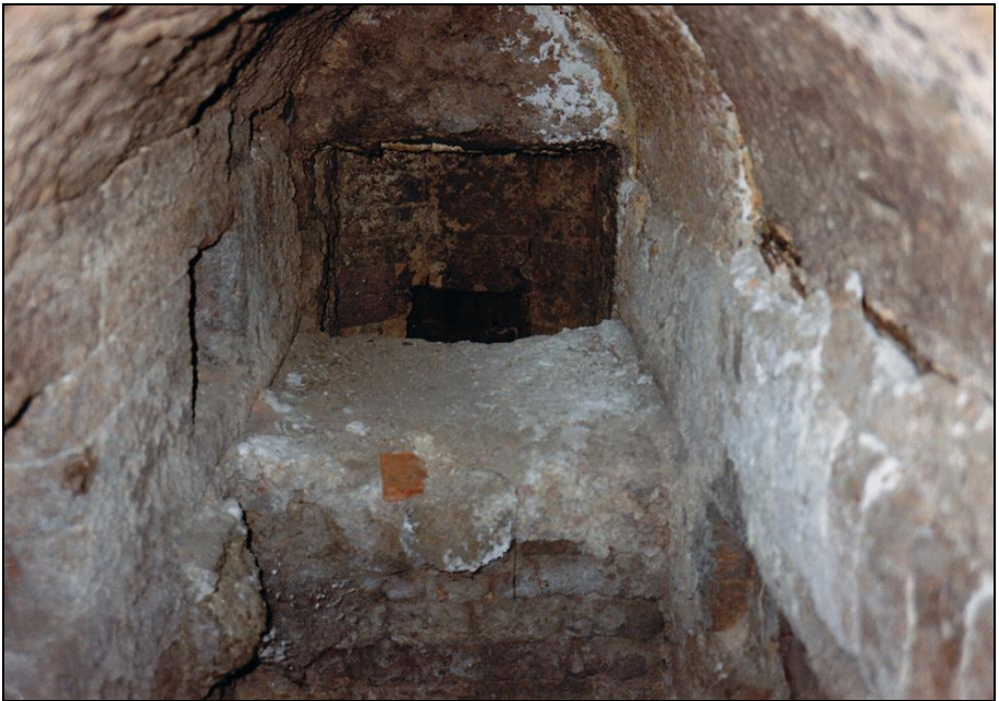
Photograph 25: Right-hand muffle: rear wall with opening for the flue gas.
