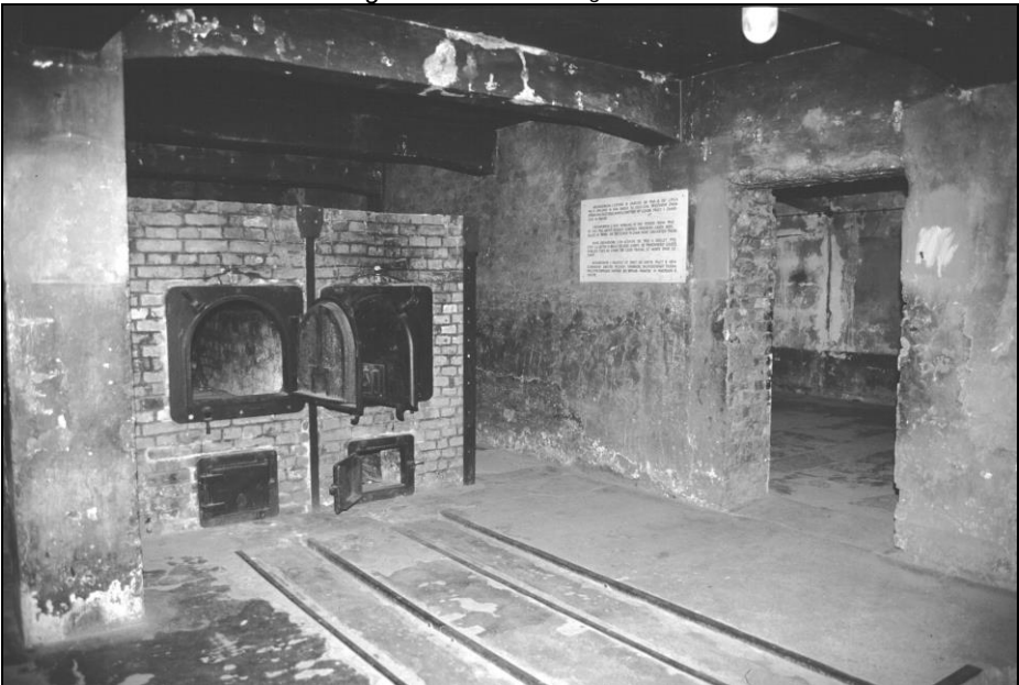
Document 29: Auschwitz, old crematorium, second cremation furnace (reconstructed by the Poles) and current access opening to the former morgue (equally created by the Poles). © Fredrick Töben 1997
