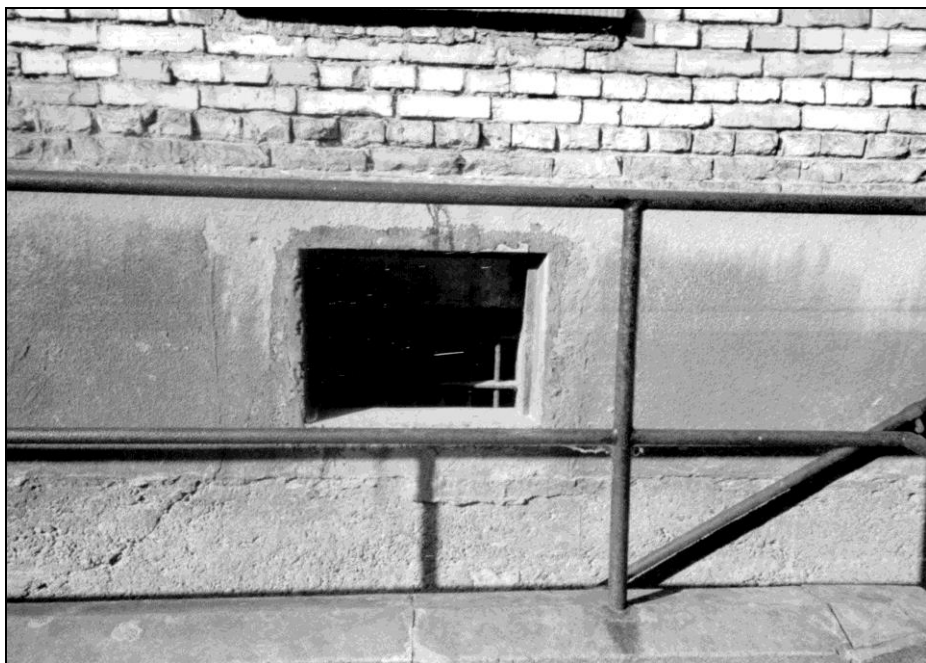
Photo 25: Block 11, outside, wall facing NNE, window of cell no. 14.
