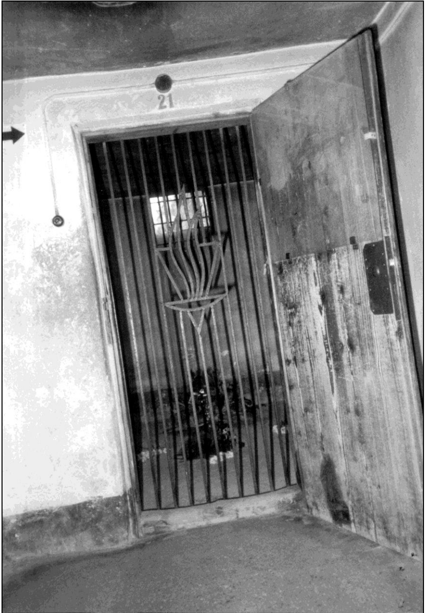
Photo 17: Block 11, inside, Bunker, right side, cell no. 21.
