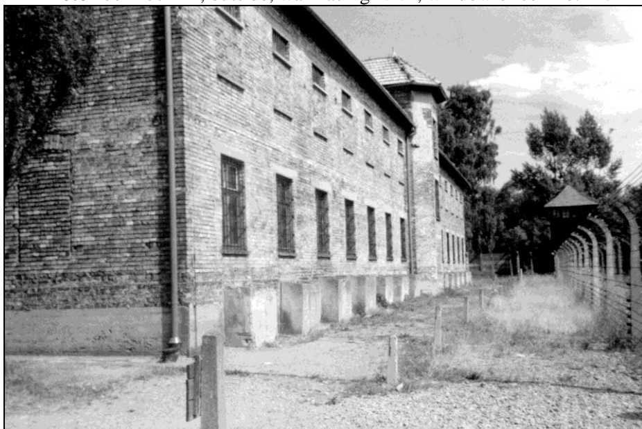
Photo 26: Block 11, outside, wall facing SSW, concrete covers surrounding the windows of the Bunker cells.
