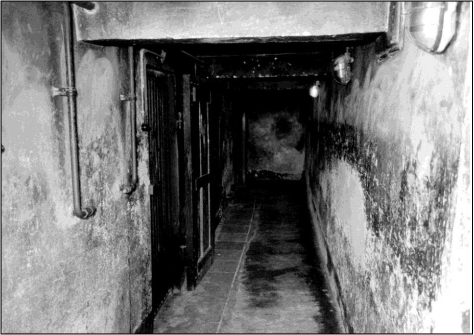
Photo 18: Block 11, inside, right side, left-side lateral corridor (cells nos. 17-20).
