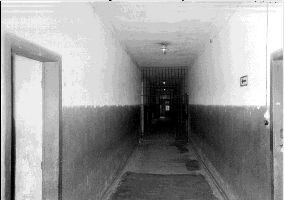
Photo 7: Block 11, inside, ground floor, hallway seen from the opposite side toward the entrance door.
