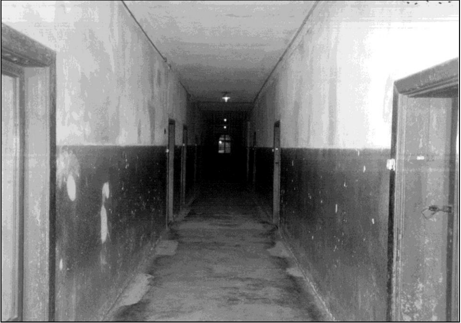
Photo 6: Block 11, inside, ground floor, hallway seen from the entrance.
