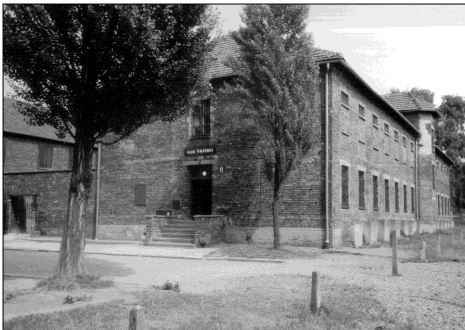
Photo 4: Block 11, outside, walls facing NE and SSW.
