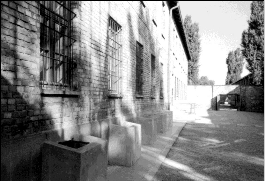
Photo 22: Block 11, outside, wall facing NNE, concrete covers surrounding the windows of the Bunker cells.
