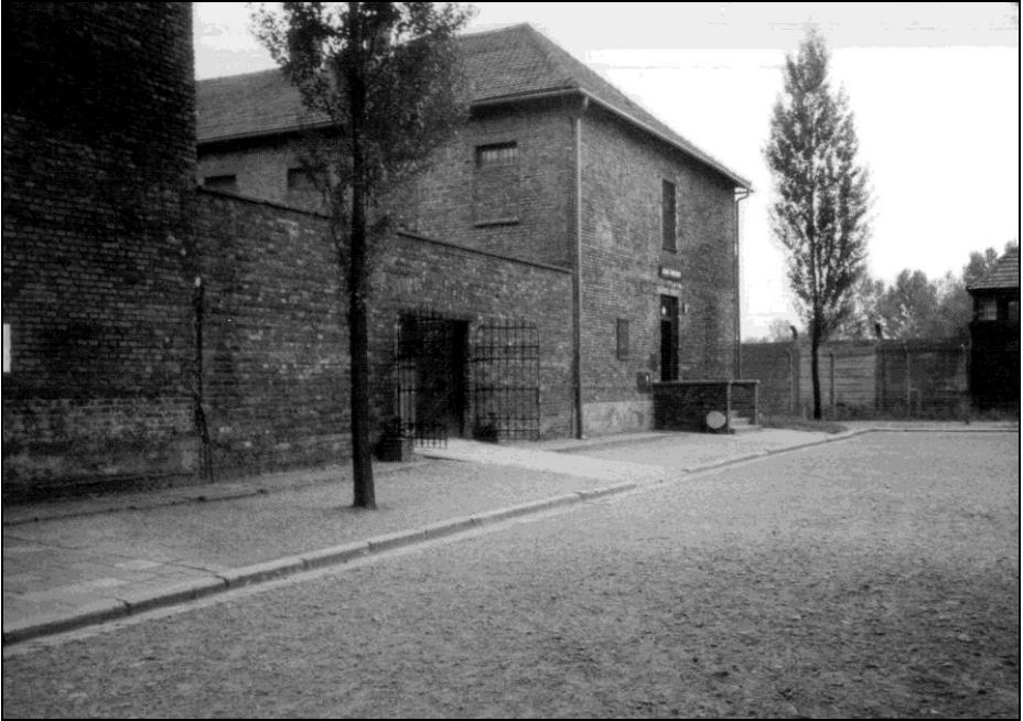
Photo 3: Block 11, outside, wall facing NE, wall and gate of the yard.
