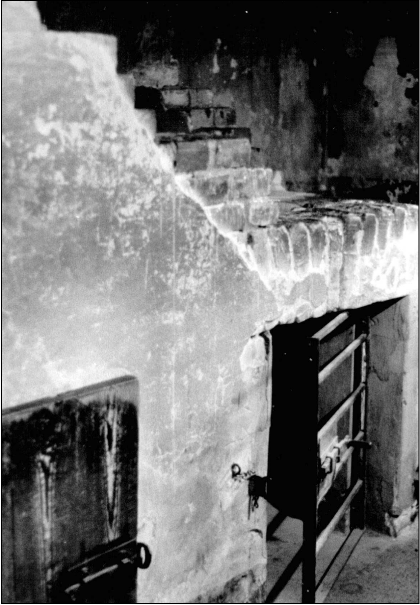
Photo 32: Block 11, inside, Bunker, right side, stand-up cells.
