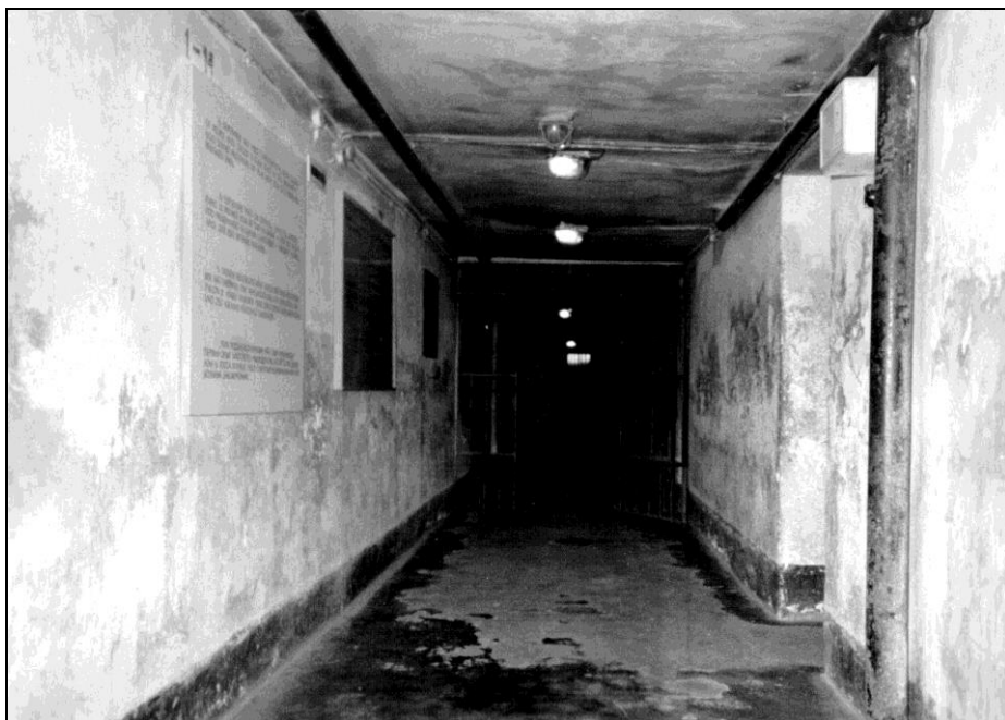
Photo 14: Block 11, inside, Bunker, right side, central hallway.
