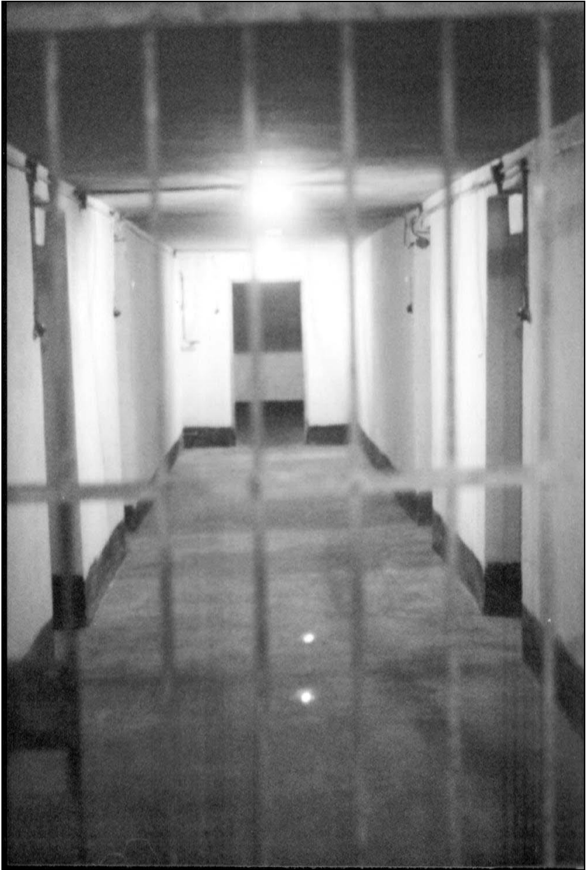
Photo 13: Block 11, inside, Bunker, left side, central hallway.
