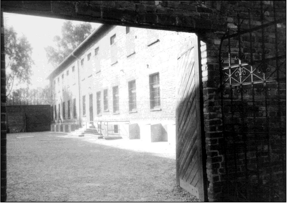
Photo 2: Block 11, outside, wall facing NNE, yard.
