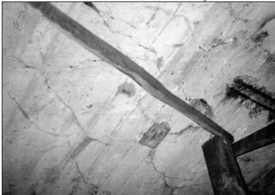
III. 10: Another one of the supporting blocks for lamps in the ceiling of Morgue 1 of Crematorium II at Birkenau. October 1991. © Carlo Mattogno.
