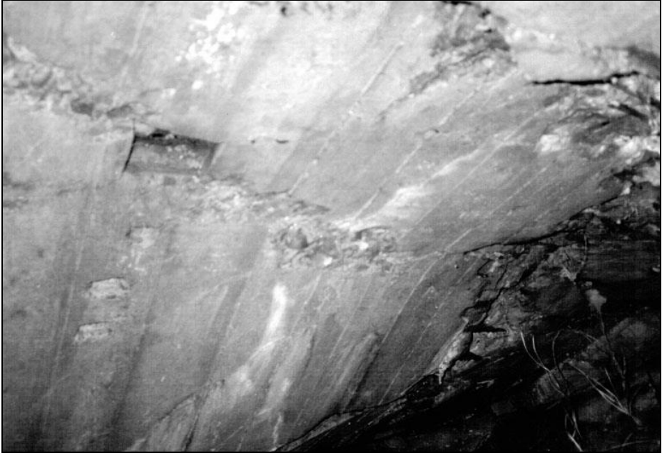
III. 11: Recess in the concrete ceiling of Morgue 1 of Crematorium II at Birkenau for a supporting block for the lamps. July 1992. © Carlo Mattogno.
