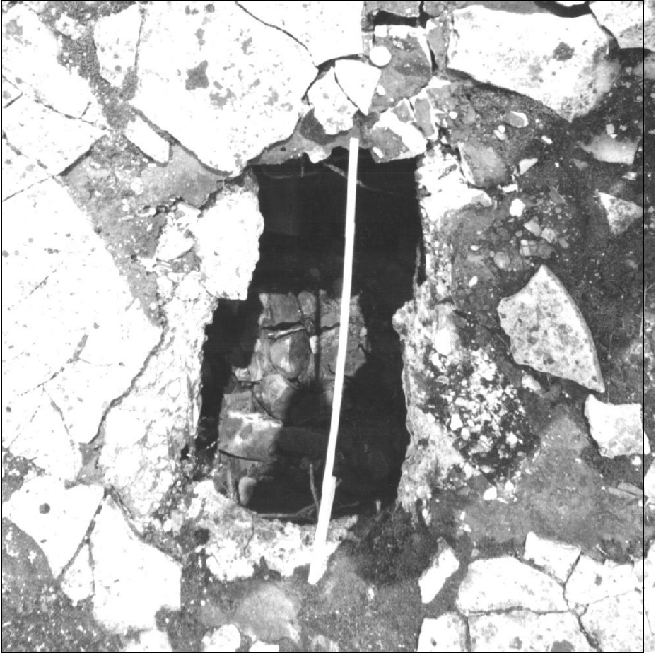
III. 18: Concrete roof of Morgue 1 of Crematorium II in Birkenau. Provan's opening 2 in August 1997. © Carlo Mattogno
