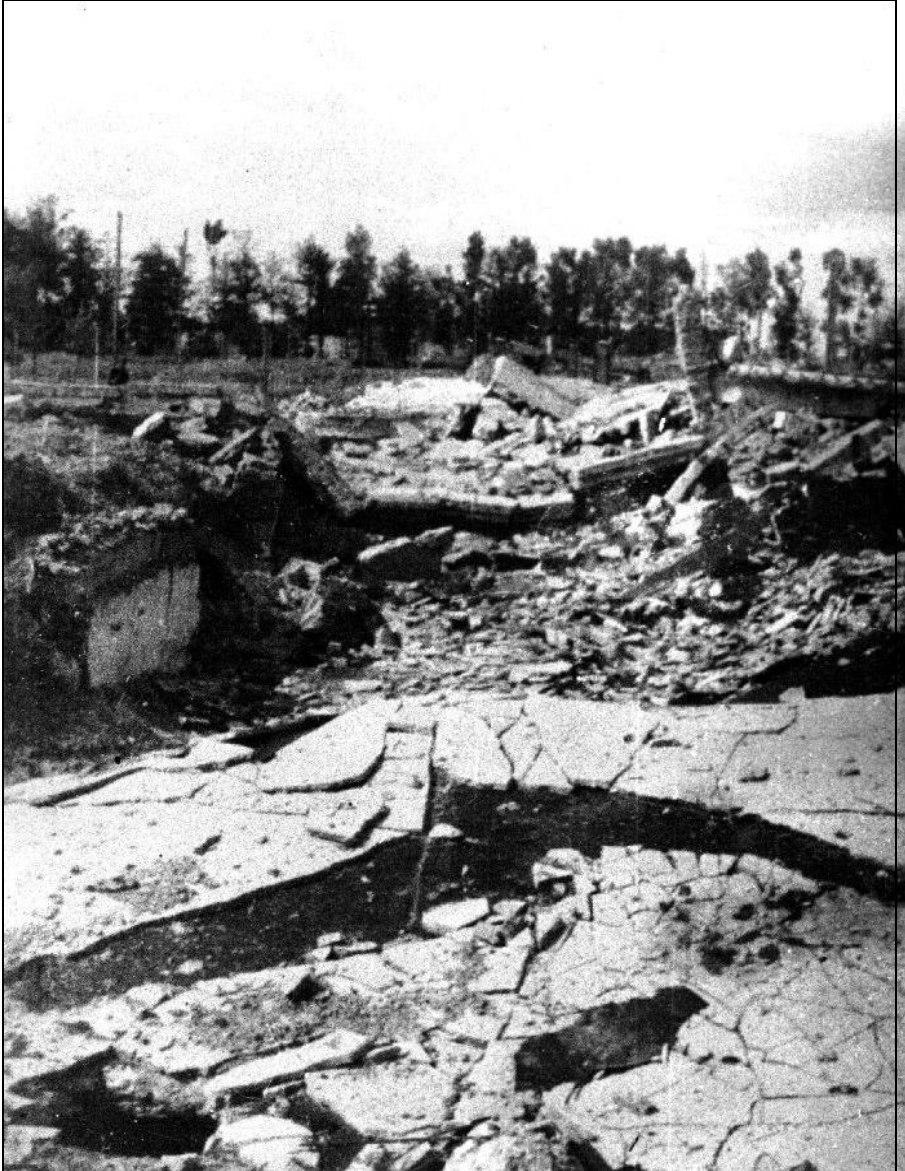
III. 5: The reinforced concrete roof of Morgue 1 of Crematorium II in Birkenau in June/July 1945. Photo by Stanislaw Kolowca.
