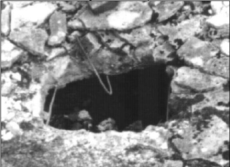
III. 28: Concrete roof of Morgue 1 of Crematorium II in Birkenau. Provan's opening 7 in August 2000. © Carlo Mattogno
