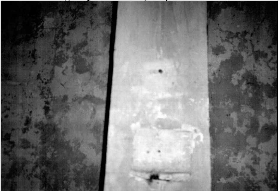
III. 12: Morgue of Crematorium I at Auschwitz. One of the blocks set into the center of the supporting beam of the ceiling. October 1991. © Carlo Mattogno.
