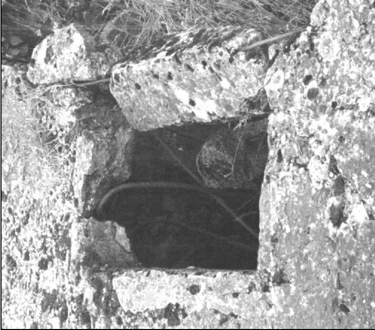
III. 13: Ceiling of the furnace room of Crematorium III. Second ventilation opening (seen from the west). June 1990. © Carlo Mattogno
