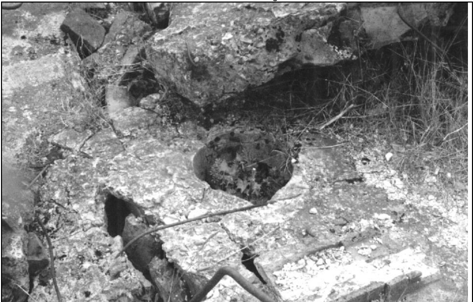
III. 11: Round opening for the pipe of the ventilation through the reinforced concrete roof of Morgue 2 of Crematorium II in Birkenau. October 1991. © Carlo Mattogno
