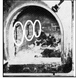
III. 2: Openings in walls of center muffle of Buchenwald triple-muffle furnace (=Birkenau furnaces, highlighted with white ellipses). 10
