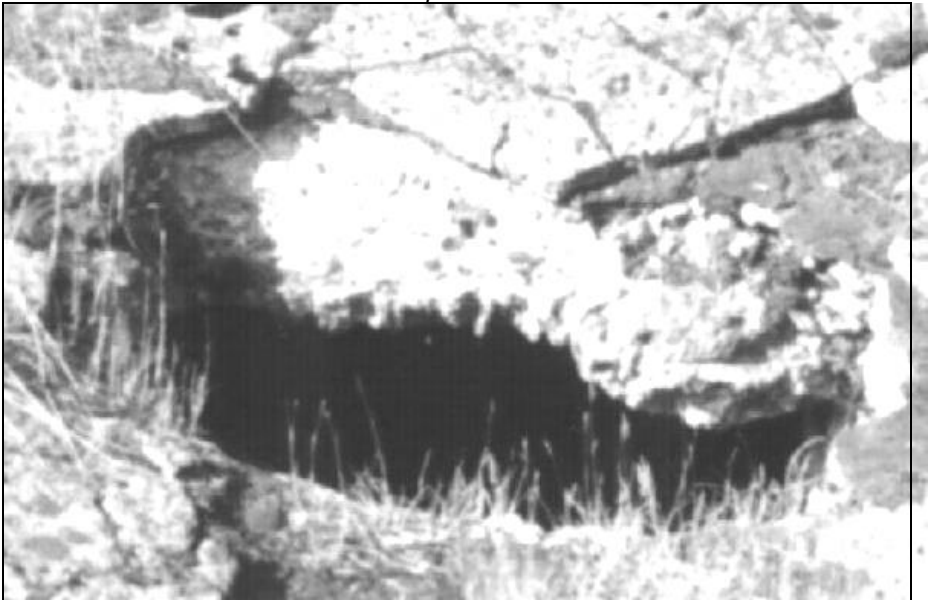
III. 20: Concrete roof of Morgue 1 of Crematorium II in Birkenau. Provan's opening 2 in July 1992. © Carlo Mattogno
