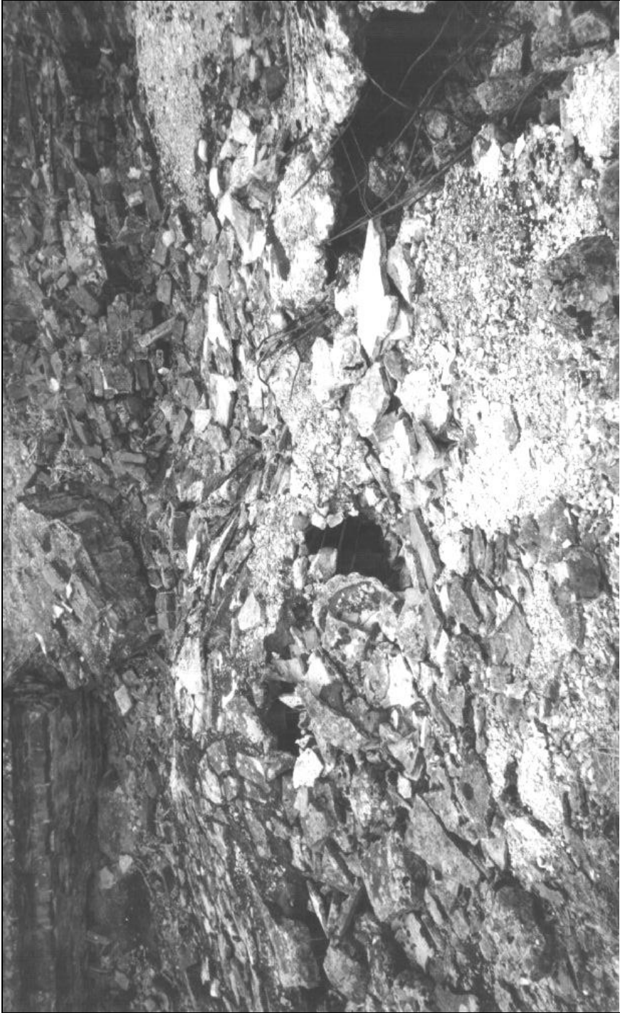
III. 34: Concrete roof of Morgue 1 of Crematorium II in Birkenau in August 2000. Provan's opening 8 (in the center) and continuation of crack (see photo 33), of which opening 8 is a part. © Carlo Mattogno
