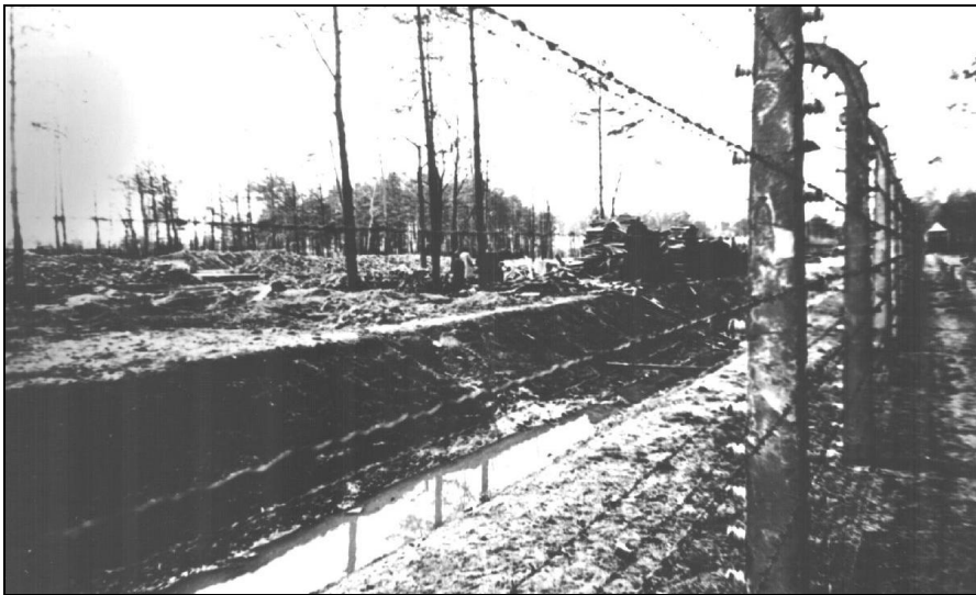
Fig. 5: Drainage ditch running north of Crematorium V.
