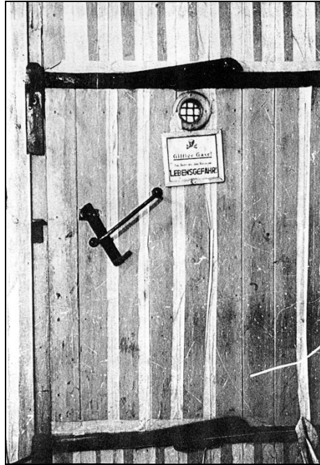
III. 124: Makeshift airtight wooden door of a delousing chamber in Auschwitz with peephole and metal grill in front. We are told that this is what airtight doors of homicidal “gas chambers” looked like. Note the flimsy latch!
