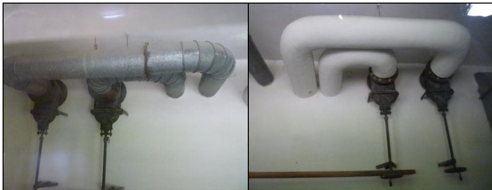
III. 24: Thick pipes in the room behind and in the area above the Dachau “gas chamber.”
