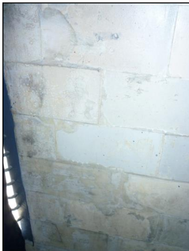
Ill. 23: Newly added tiles, or rather, fake tiles, around the introduction chutes.
