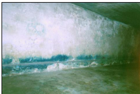
III. 89: Zyklon-B delousing installation, Chamber III (east wall), of building 41 in Majdanek. (© C. Mattogno)
