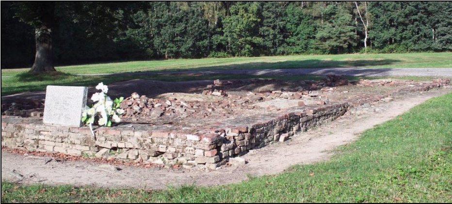
III. 111: Foundation walls of an old building, allegedly Bunker 2, west of the Zentral-sauna in Birkenau.
