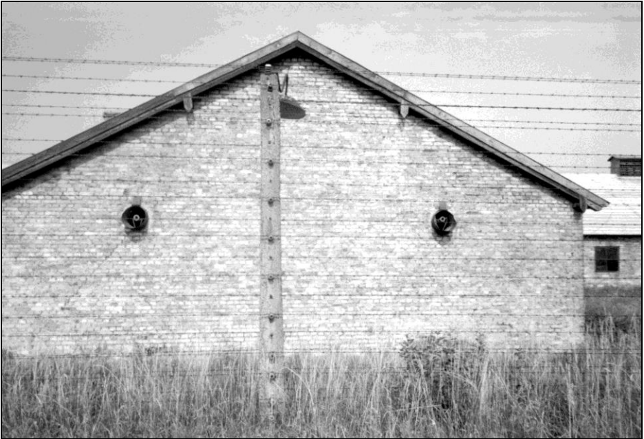
1. Birkenau, BW 5b, round openings for placement of ventilators in the outside wall of the gas disinfestation chamber. July 1992, © Carlo Mattogno.
