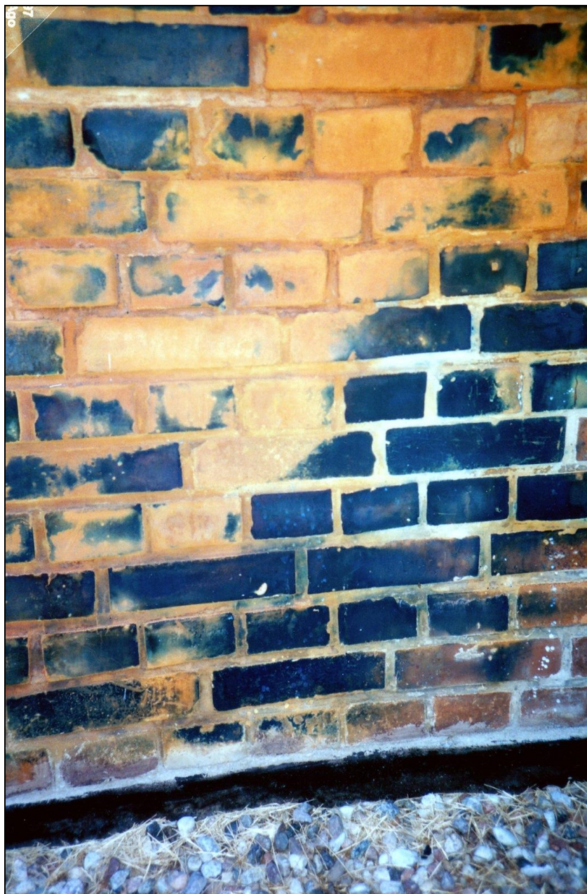
Photo 16: Delousing chamber at Stutthof, east side, exterior. The brick exhibits the typical blue pigmentation caused by iron cyanide.
