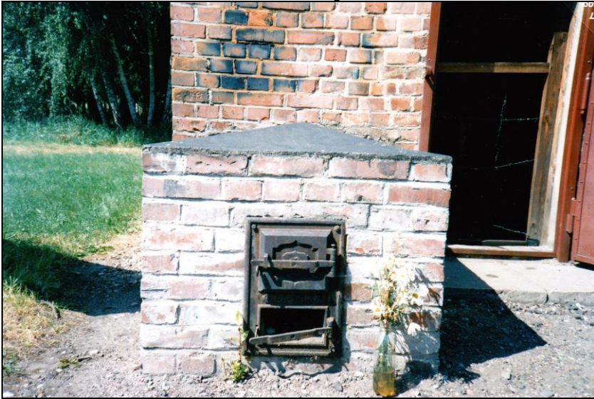
Photo 6: Delousing chamber at Stutthof, viewed from the south. The stove was used to heat the air inside the delousing chamber. Above: the fire door. Below: the ash door. © Carlo Mattogno
